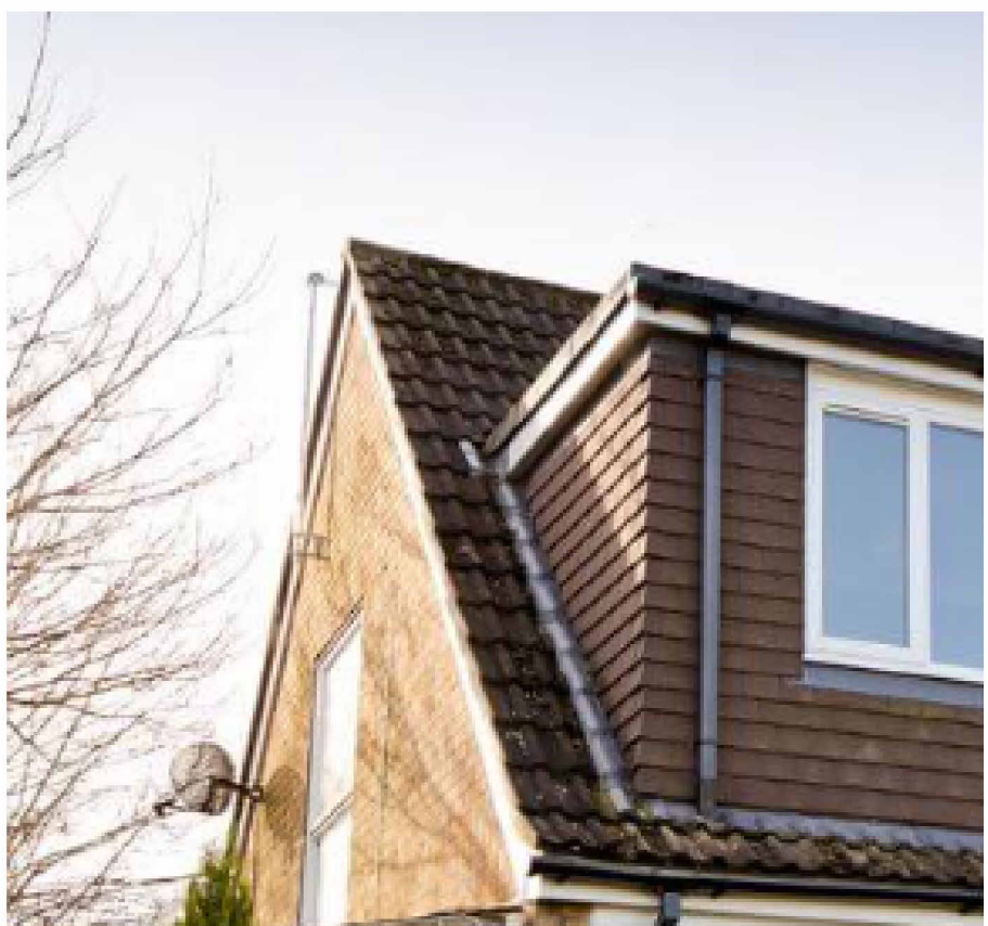
example of roof and dormer tiles
