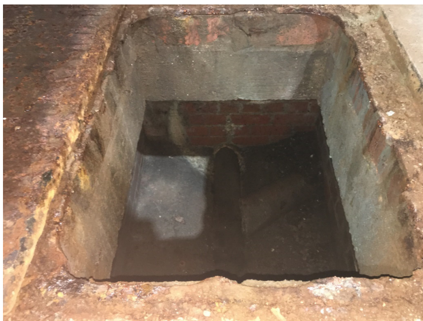
Figure 5.0 – Southern warehouse manhole chamber
