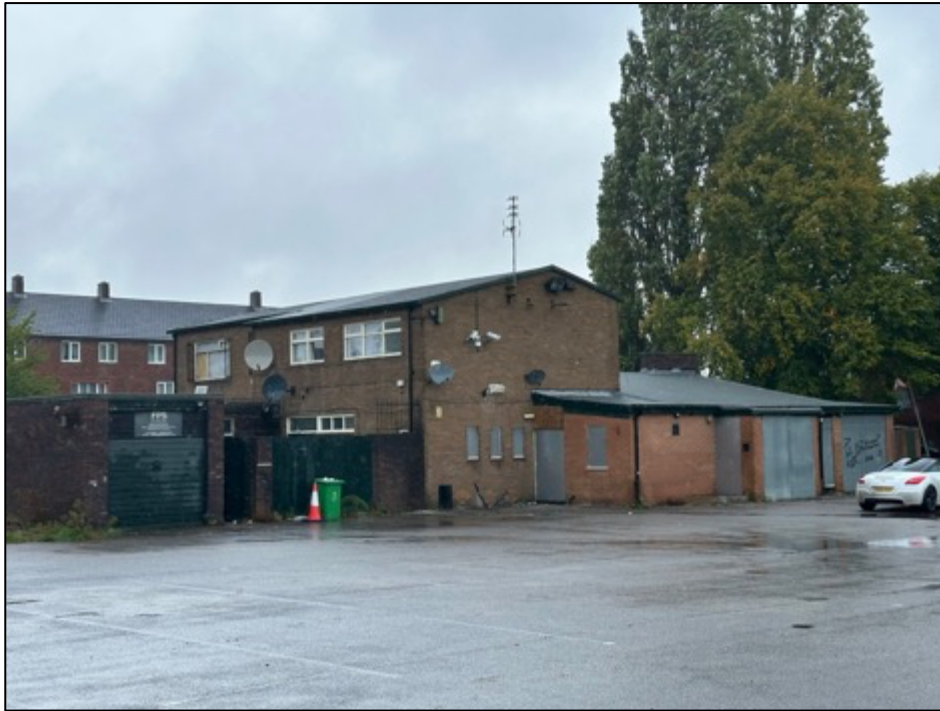
Photograph 1; An external view from the southern side of the building, clearly showing the composition. The building features several single storey extension sections, all sections feature a felt external roof.
