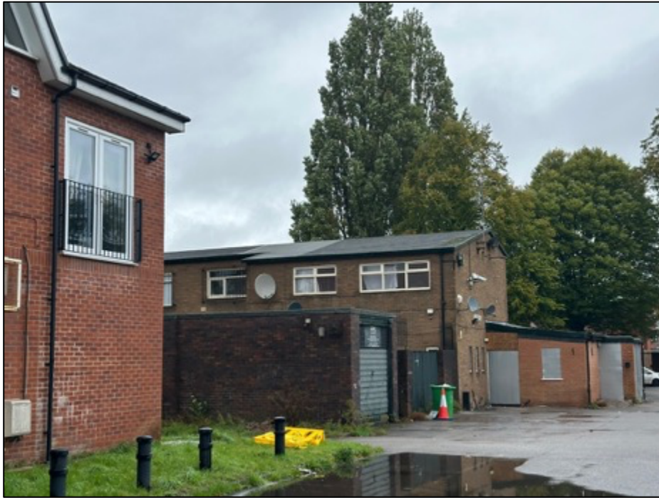
Photograph 9; A distant view of the external felt roof. The roof is in good condition considering the age and composition.
