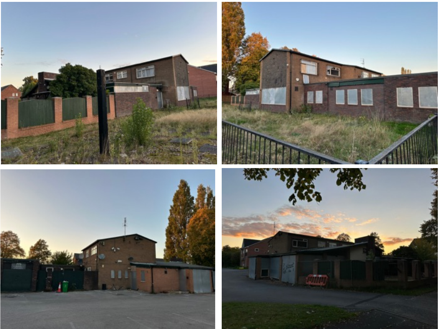
Figure 2: Surveyor and Thermal Imaging Camera Viewpoints.
