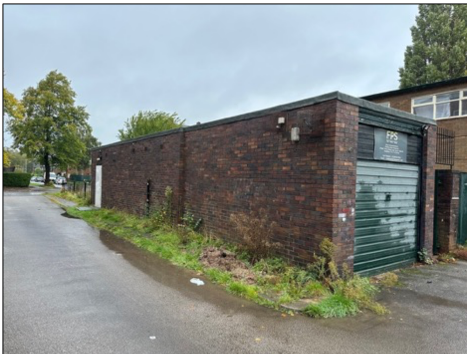
Photograph 3; A view of the attached flat roof section with corrugated roller door. A slight linear buffer of modified grassland, featuring common thistle and stinging nettle.
