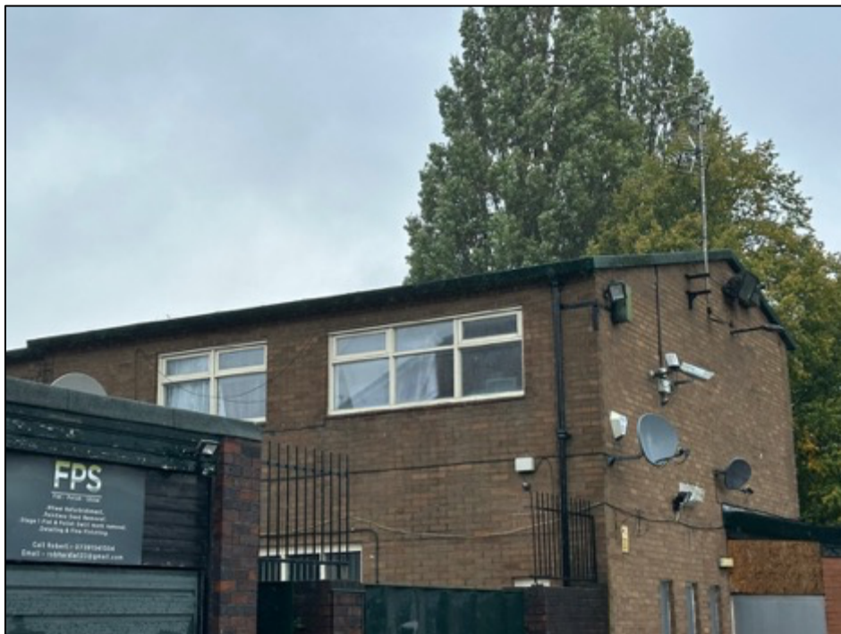
Photograph 2; View of the main section of the building, showing the two-storey base of the former pub. The external brick walls are well-structured and in good condition.
