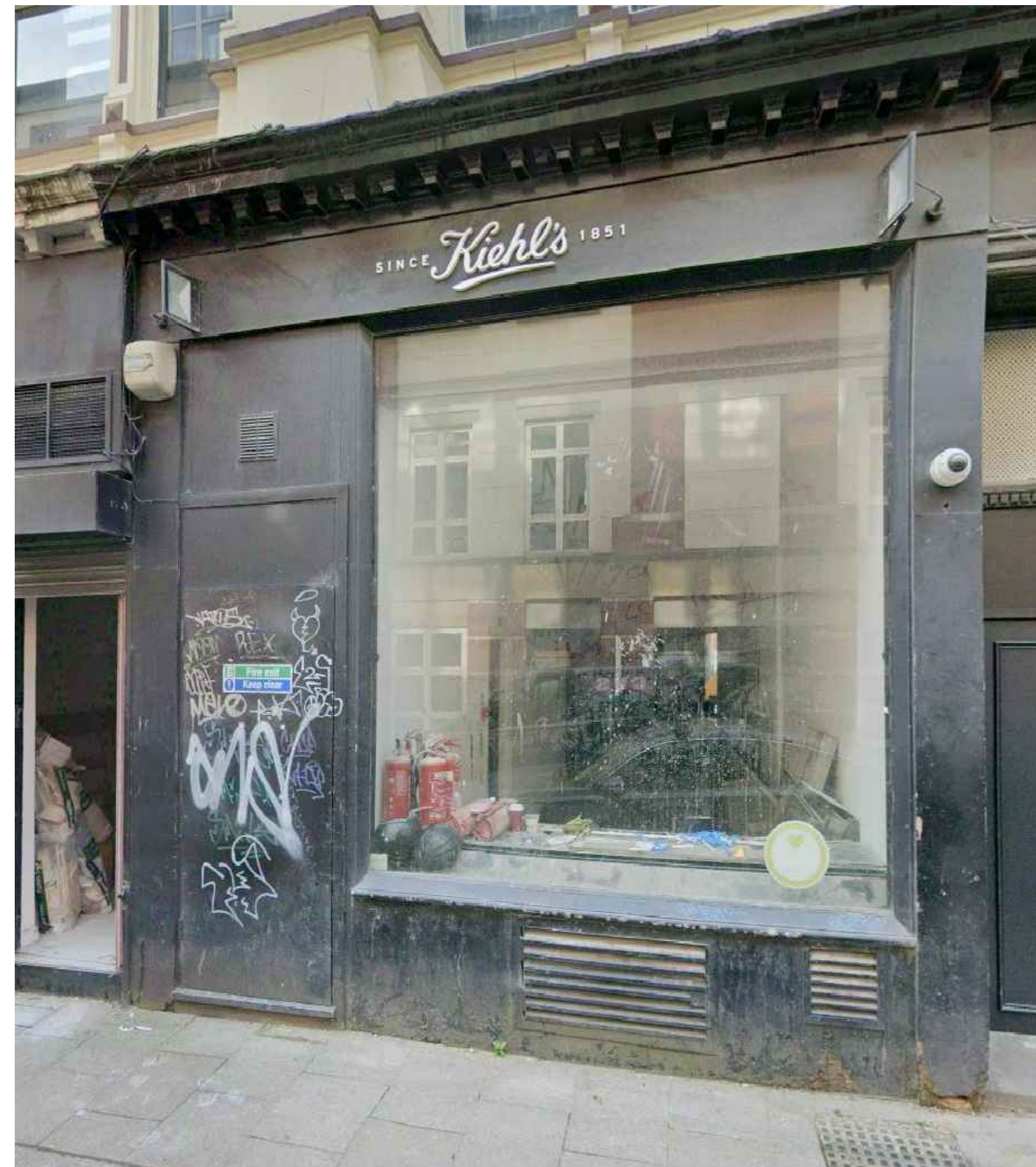
02 EXISTING PHOTO - S.KING ST.
