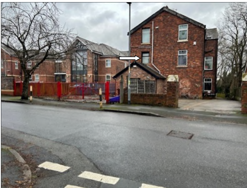
View of application site from Windsor Rd / Elisma Rd junction
