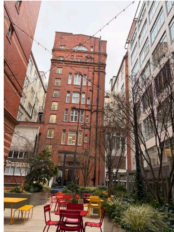
View towards the rear of Broadhurst House from the courtyard with the 1960's infill on the right.
