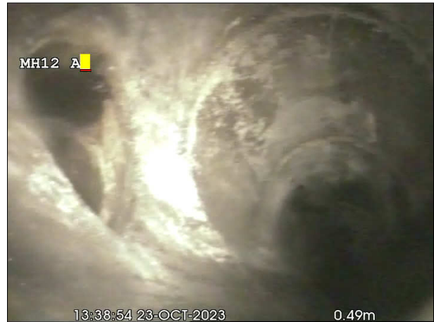
Photo: 189_4b, 00:00:00 0.5m, Junction at 09 o'clock, dia 150 mm
