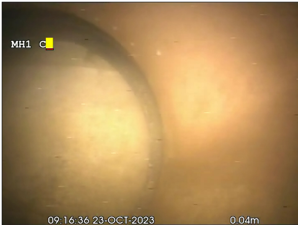
Photo: 26_4a, 00:00:00 0.3m, Finish Survey, Remark: Line capped.
