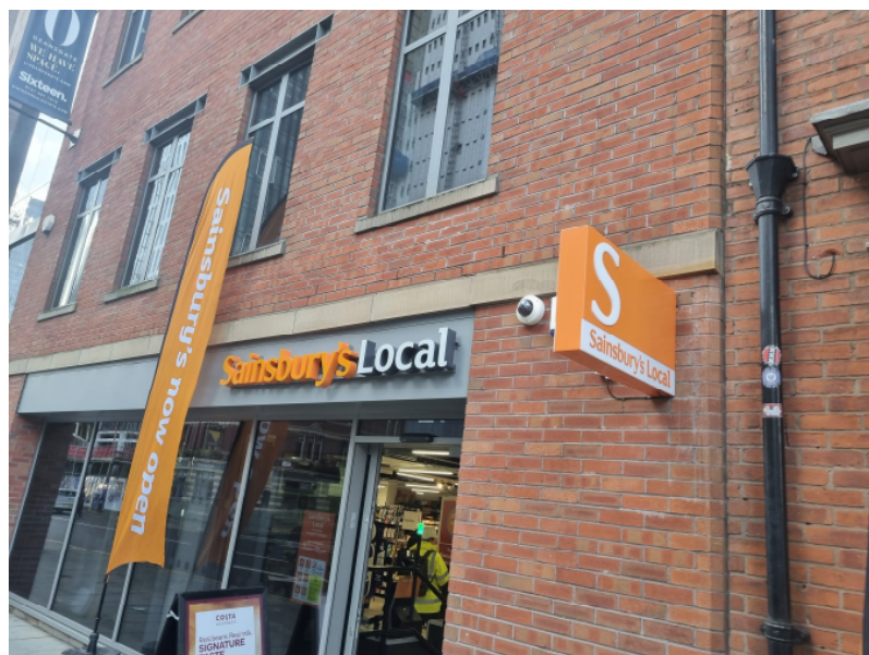
Existing site, including previously approved signage and unauthorised projecting sign.
