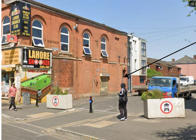
Figure 4. – Mayford rd loading area
