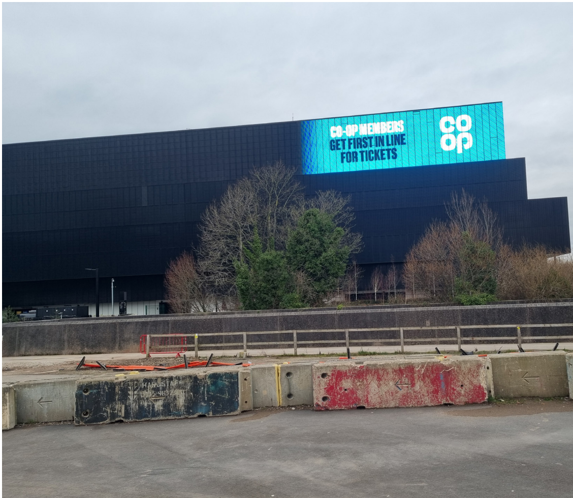
Looking towards Co-op Live from site - day
