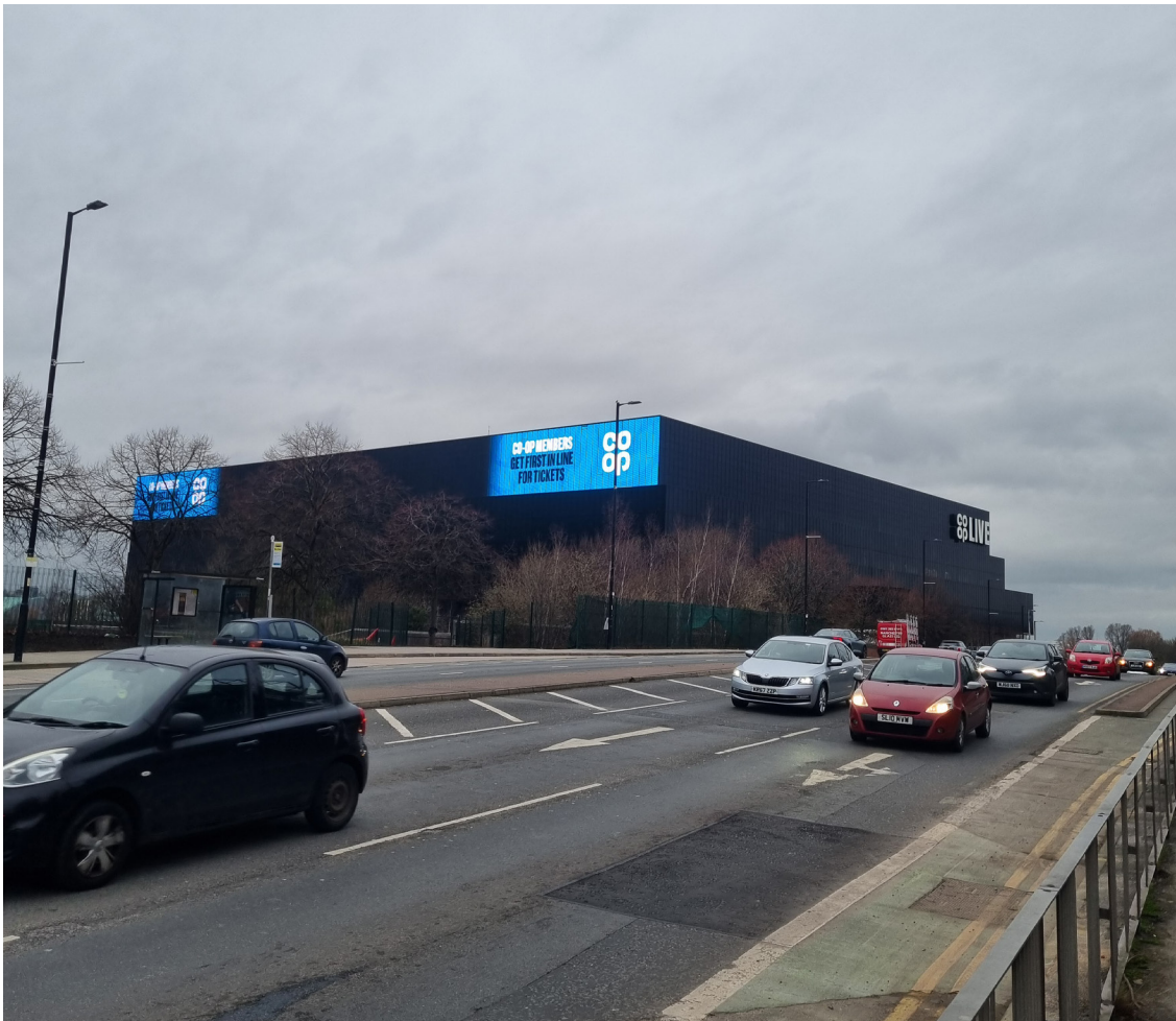
Looking towards Co-op Live from Alan Turing Way - night
