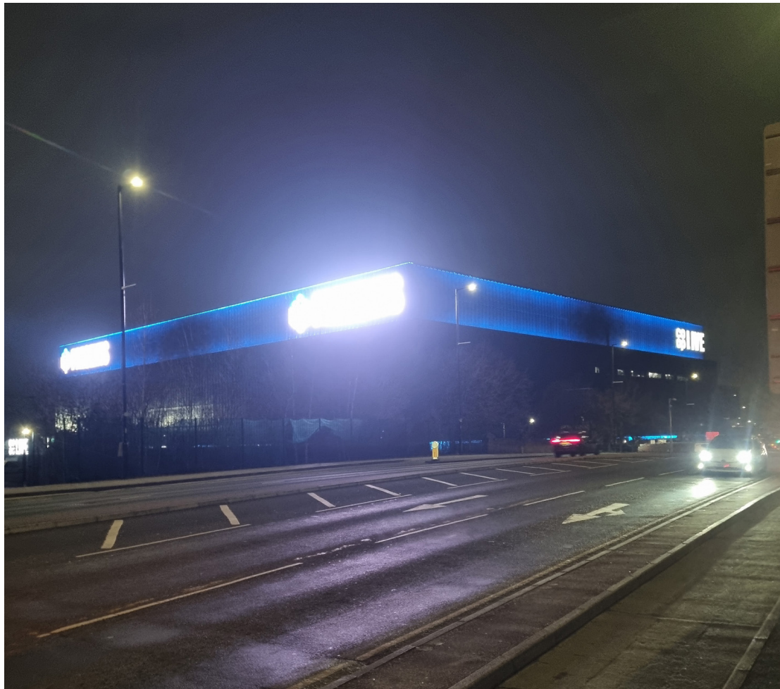
Looking towards Co-op Live from Alan Turing Way - day
