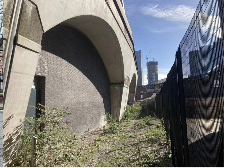
2. Rear infill of 121 Water Street.
