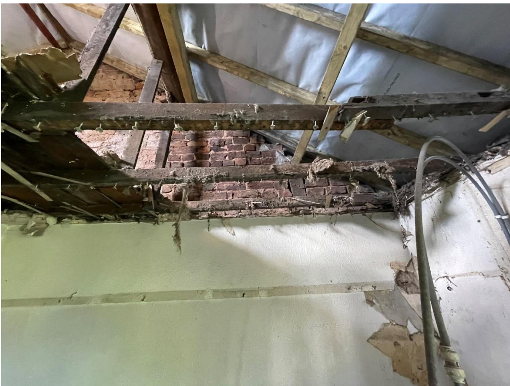
PHOTO 14 – ADDITIONAL TIMBER ROOF PURLINS INSTALLED IN THE PAST
