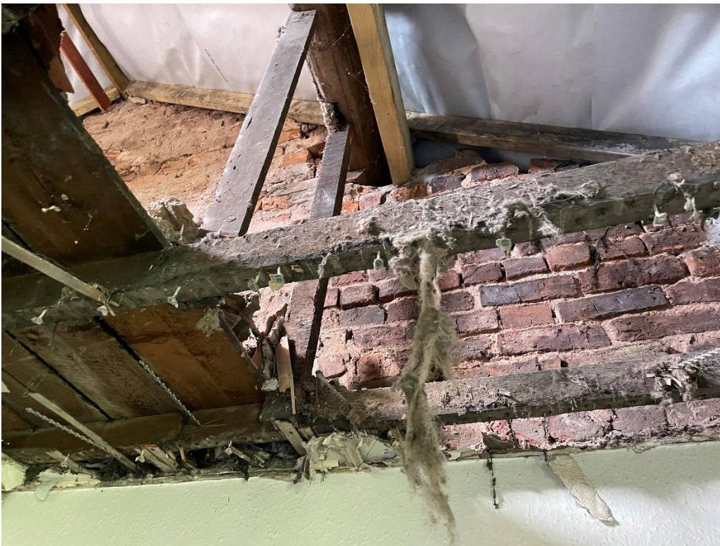
PHOTO 16 – STEEL HELI-BAR TIES INSTALLED THROUGH GABLE WALL IN THE PAST
