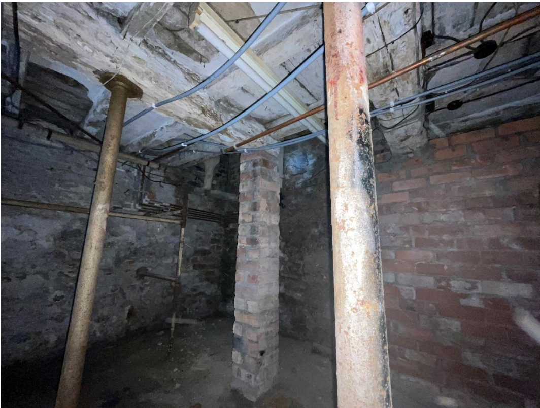
PHOTO 11 – STEEL PROPS AND MASONRY PIER SUPPORTING ORIGINAL TIMBER FLOOR BEAMS
