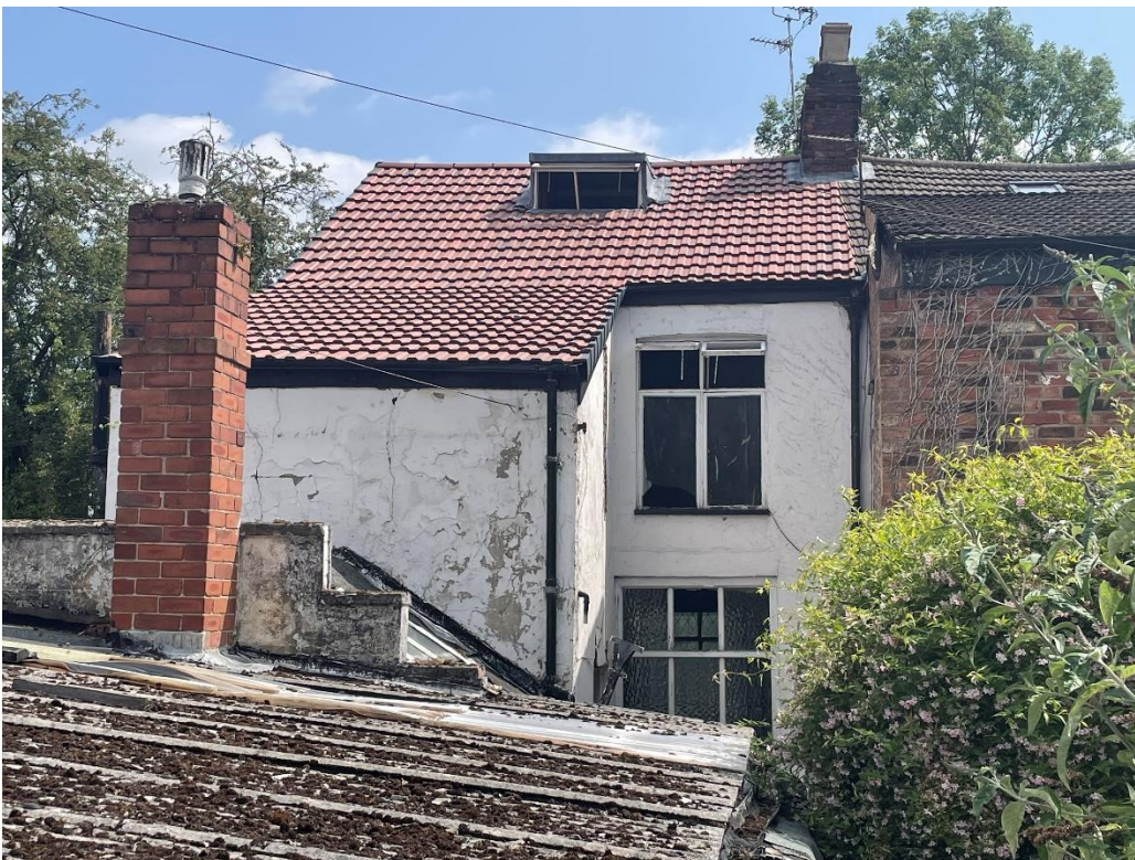
PHOTO 2 – REAR ELEVATION OF MAIN BUILDING WITH MODERN TILED ROOF COVERINGS & DORMER
