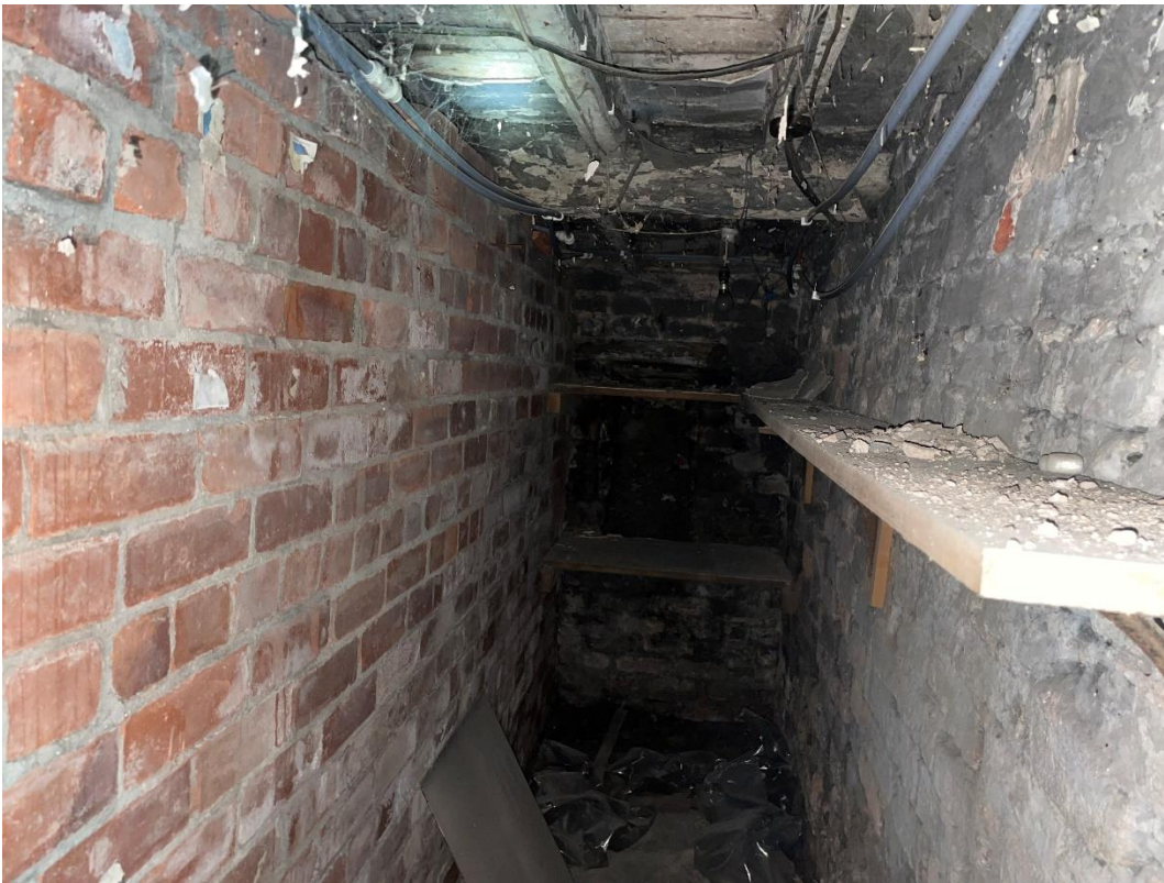
PHOTO 15 – NEW 215MM BRICKWORK SKIN CONSTRUCTED ADJACENT TO BASEMENT SIDE WALL
