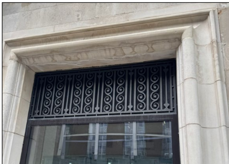
Figure 1 Decorative Grille Along Quay Street Elevation
