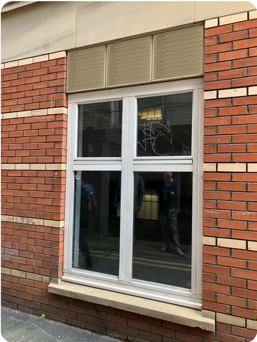
Lintel replaced with louvres - Sits in same plane as existing lintels which are recessed slightly
