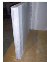
Prime & Paint like drywall
