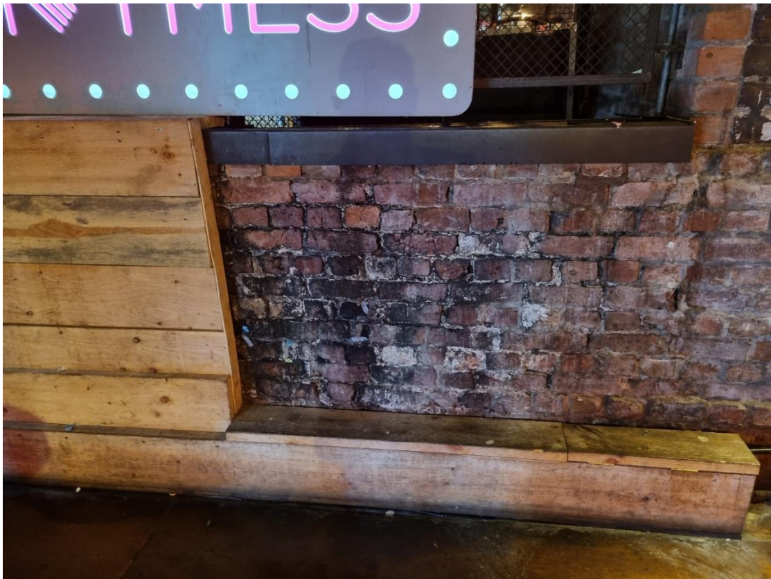
Typical water ingress to soffit
