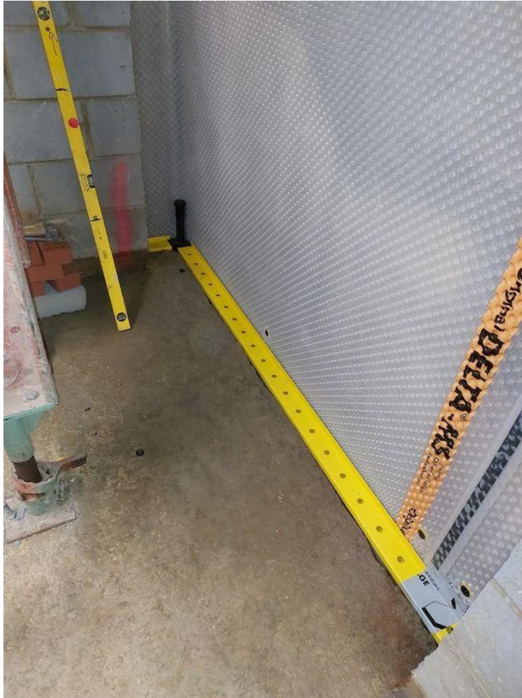
Typical Type C waterproofing membrane prior to application of a lining
