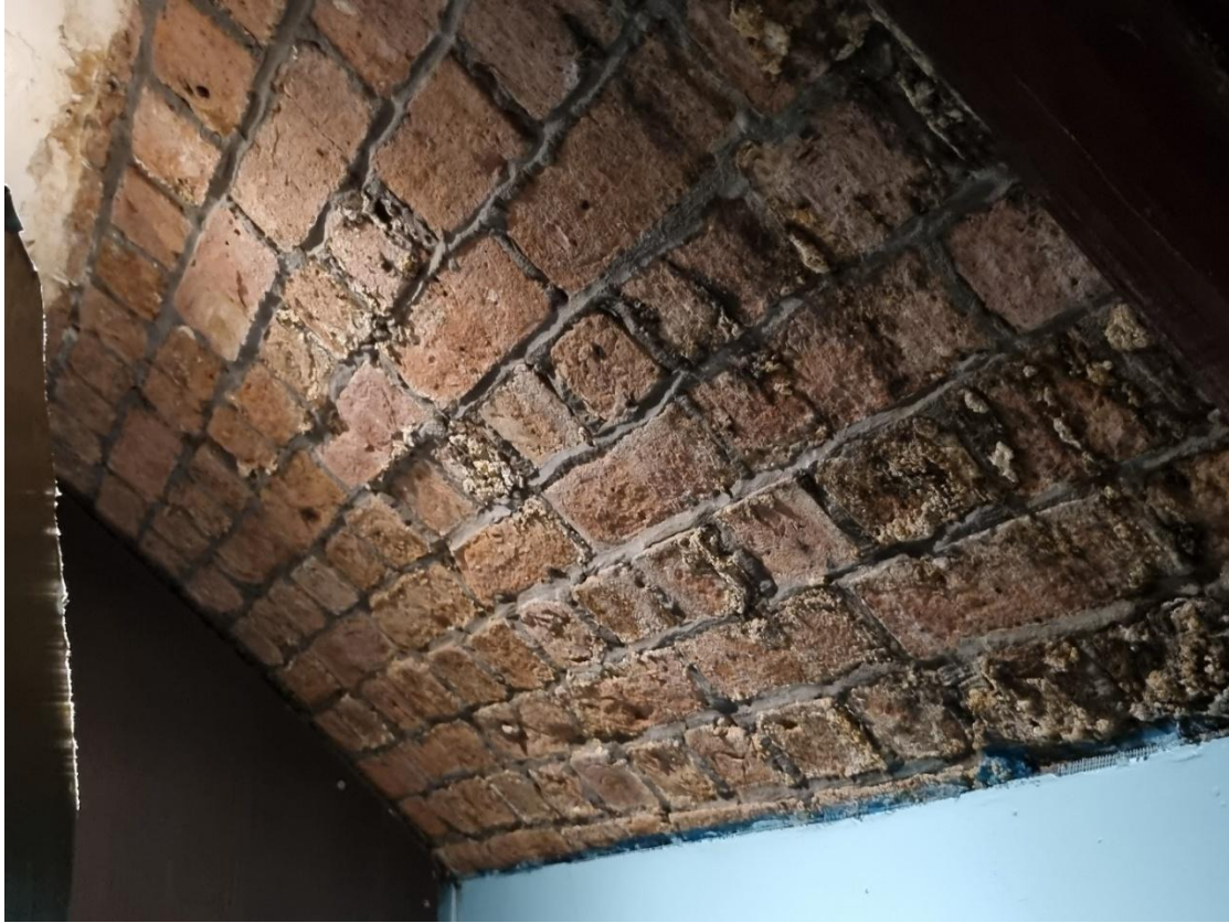
Typical water ingress to soffit
