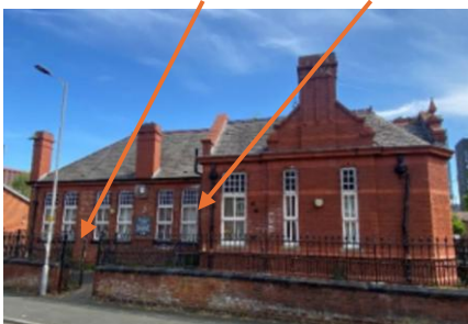
fig 1 – west elevation (barrack St) showing main gate and door
