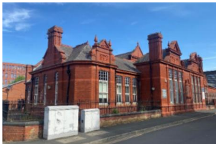
fig 2 – south elevation (quenby st) no access routes this side
