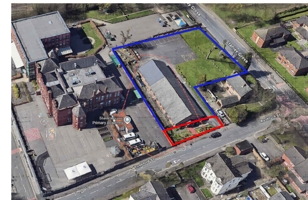
Aerial View of Site
