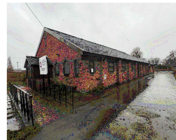
Photo of existing porch and ramp
