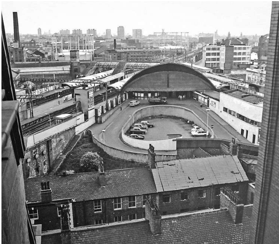
Photo of Station main access from the Refuge, picture taken by Philip Andrews
