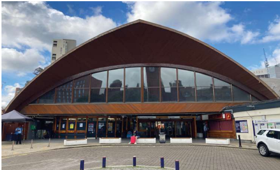
Main station access (Seed Architects Image)
