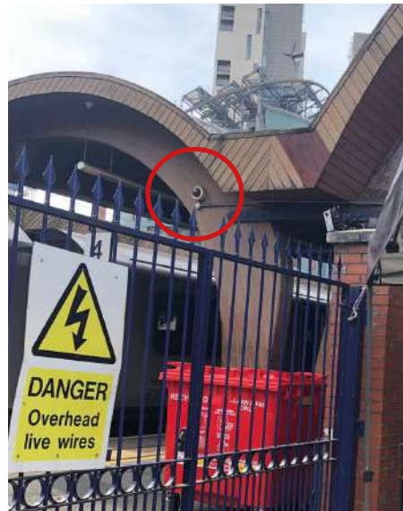
Camera on timber structural element (Seed Architects Image)
