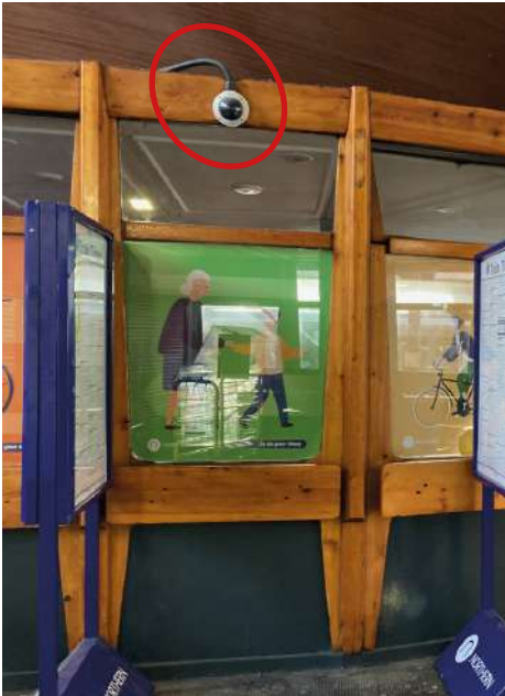
Existing device on ticket office facing the access (Seed Architects Image)
