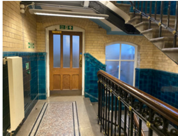
3.4.13 Ground floor stairwell
