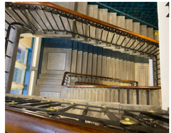
3.4.16 View from the third floor down the stair flights
