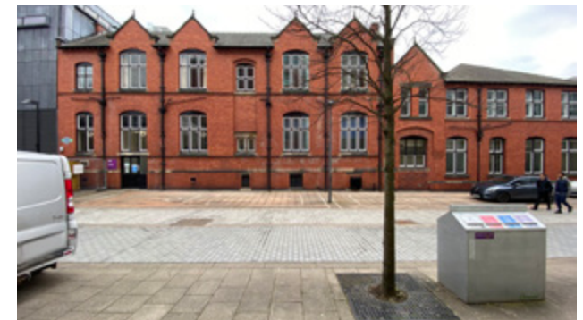
3.1.3 Frontage of the Hopkinson Memorial Wing on Bridgeford Street
