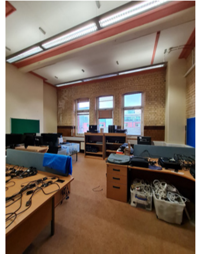
3.4.69 2.059 main space and outer wall (IBI)
