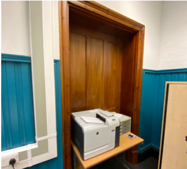
3.4.52 Extant doorway between 2.051 former lecture theatre, and 2.052, former preparation rooms
