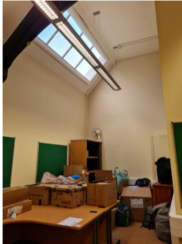
3.4.62 2.054 with later WC partition
