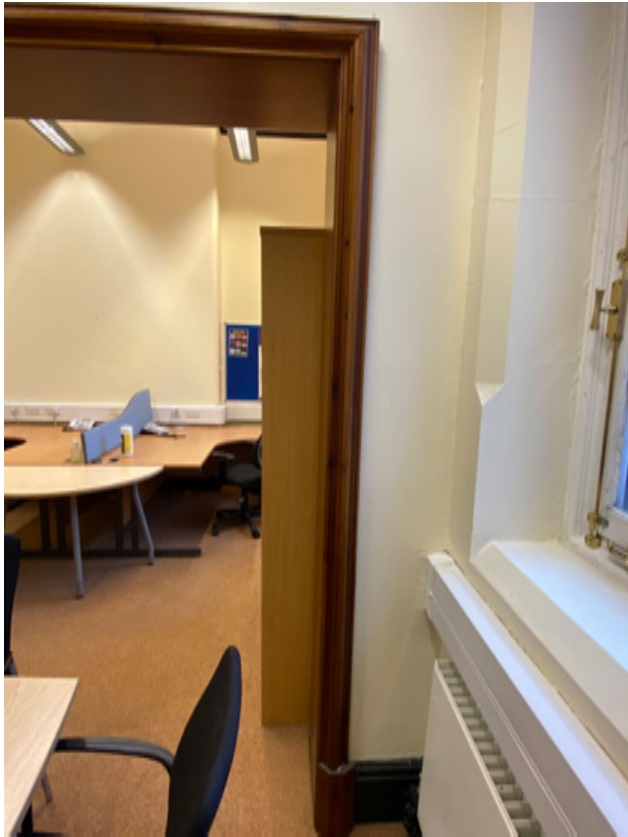
3.4.47 Open arch in Room 1.058
