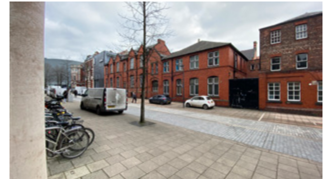
3.1.2 Southern frontage of Bridgeford Street
