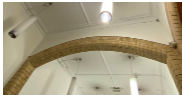
3.4.6 Exposed brick around arches in the entrance corridor
