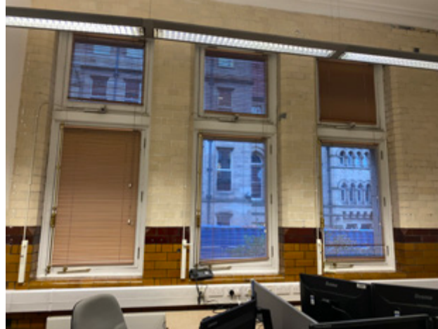
3.4.25 Glazed tiles to outer wall of G.057, with window detailing
