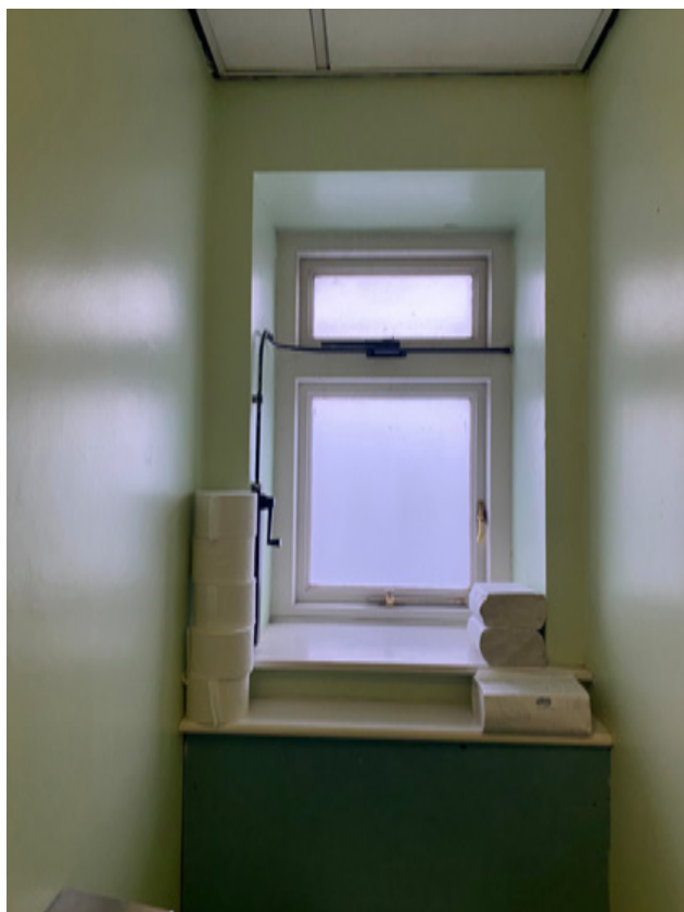
3.4.64 Room 2.056 disabled WC, projecting into 2.057
