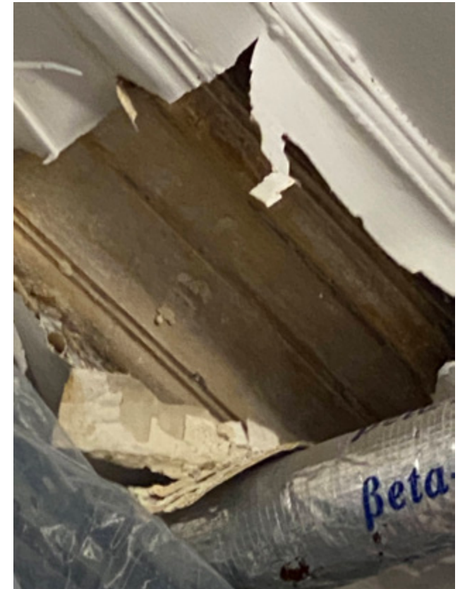
3.4.19 Cornice to the basement corridor ceiling
