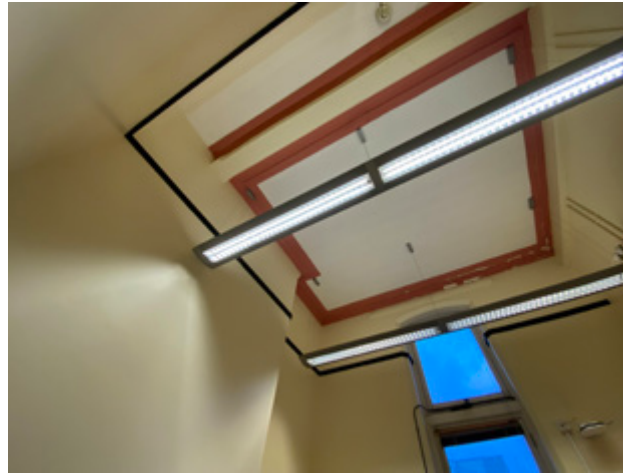
3.4.45 Ceiling of Room 1.058 truncated by the lift shaft
