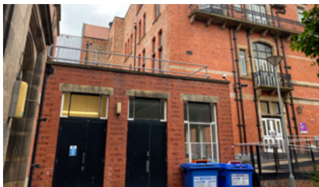
3.3.8 West return elevation as it meets the rear elevation
