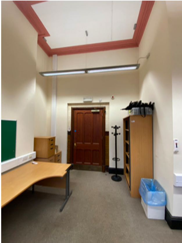
3.4.44 Room 1.057 with cornice wrapping around partition to 1.056 (storeroom)
