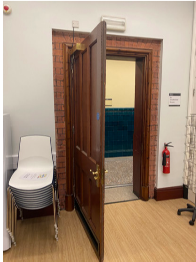
3.4.35 Brick detailing around the door in 1.053
