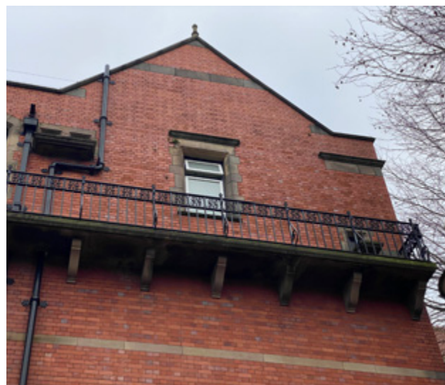
3.3.10 Closeup of the stone ledges (above the balcony) and apertures used for light experiments
