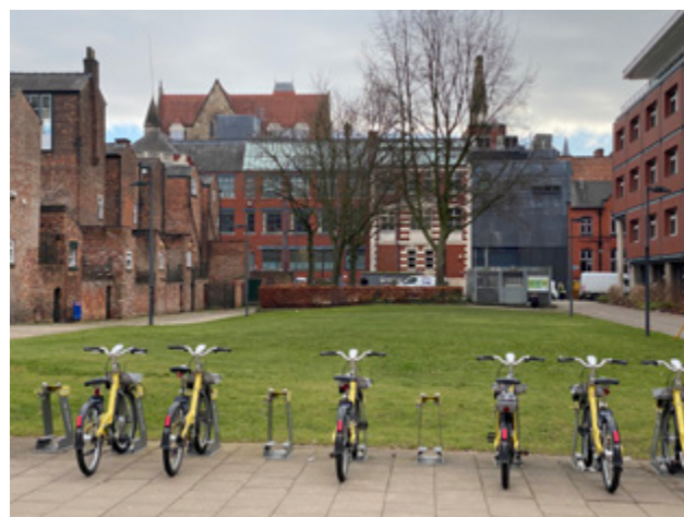
3.3.11 View of the roofscape along Bridgeford Street from University Green
