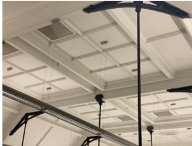
3.4.54 Ceiling detailing in Room 2.051
