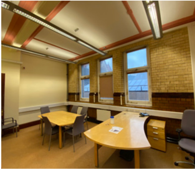
3.4.58 Room 2.052a with east elevation windows and door into 2.051
