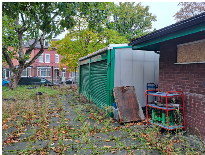
Shelter to South Elevation
