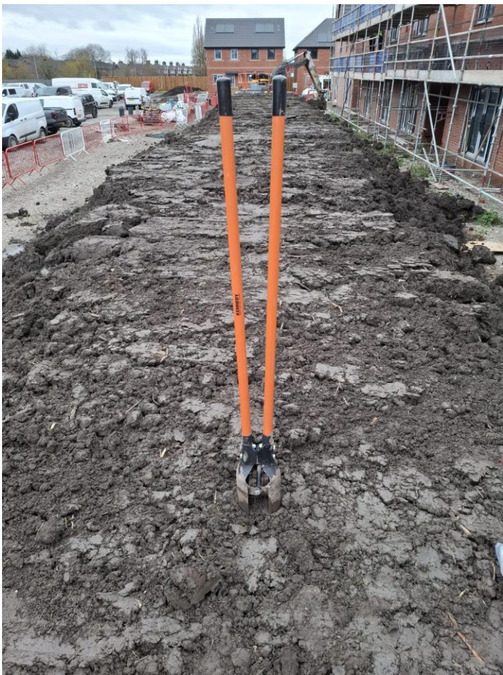
PHOTO 5: TS16-01 HOLE DIG VIEW
