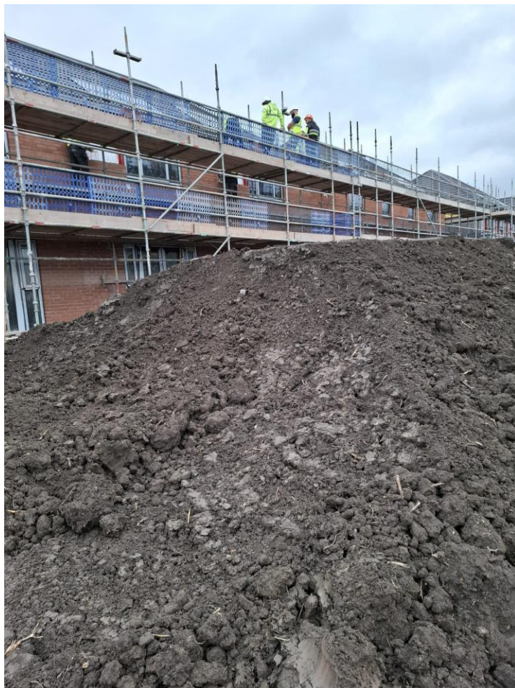
PHOTO 3: WESTERN VIEW OF STOCKPILE
