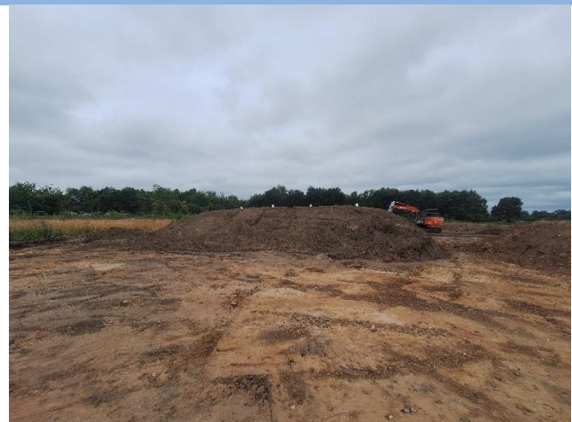
Photograph 5 – TS5 Lengthways view
