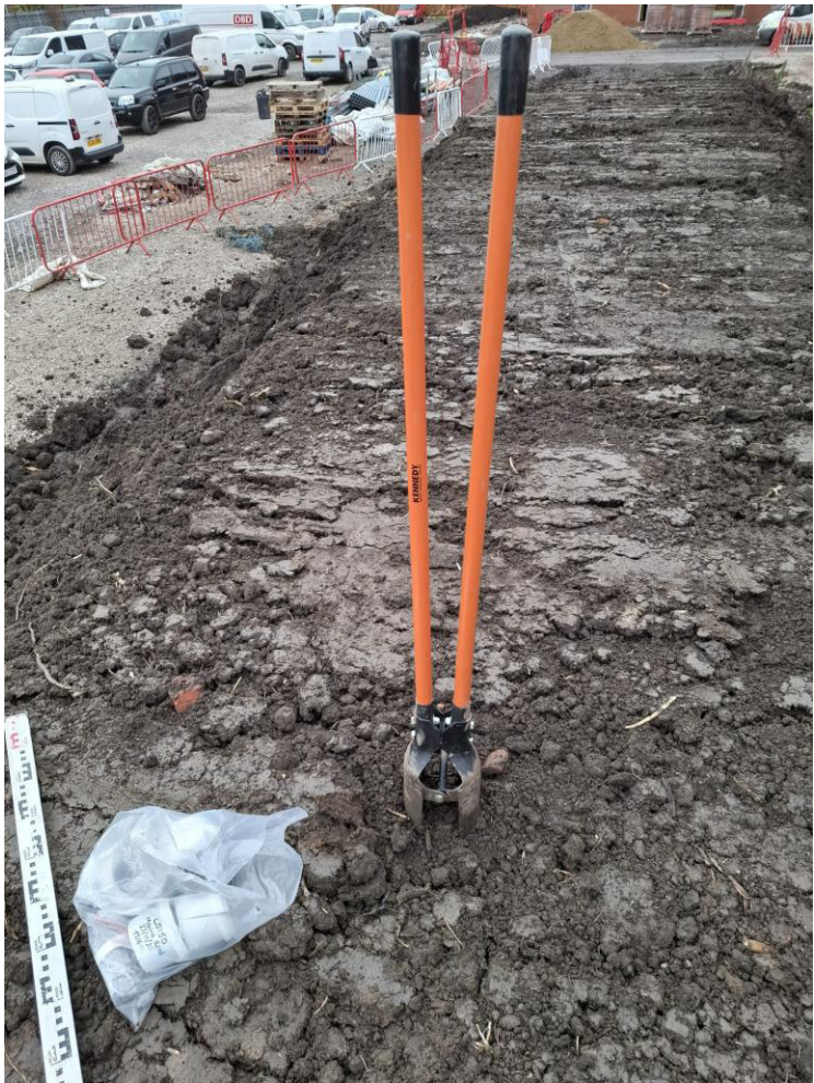
PHOTO 8: TS16-03 HOLE DIG VIEW
