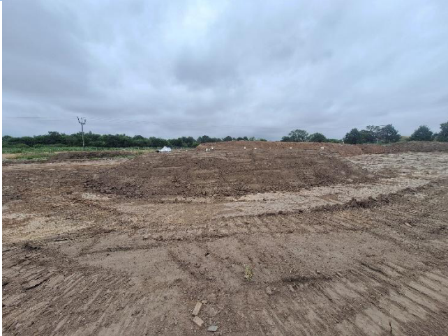
Photograph 1 – TS5 Lengthways view
