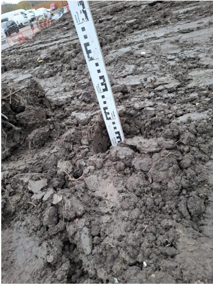
PHOTO 5: TS16-02 HOLE MEASUREMENT
