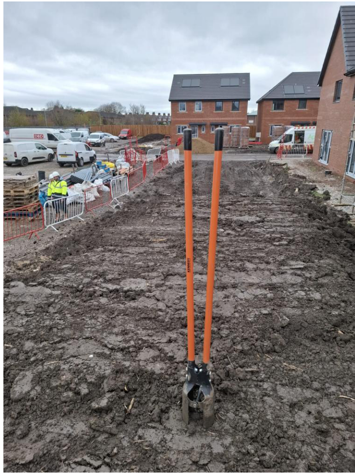
PHOTO 7: TS16-04 HOLE DIG VIEW
