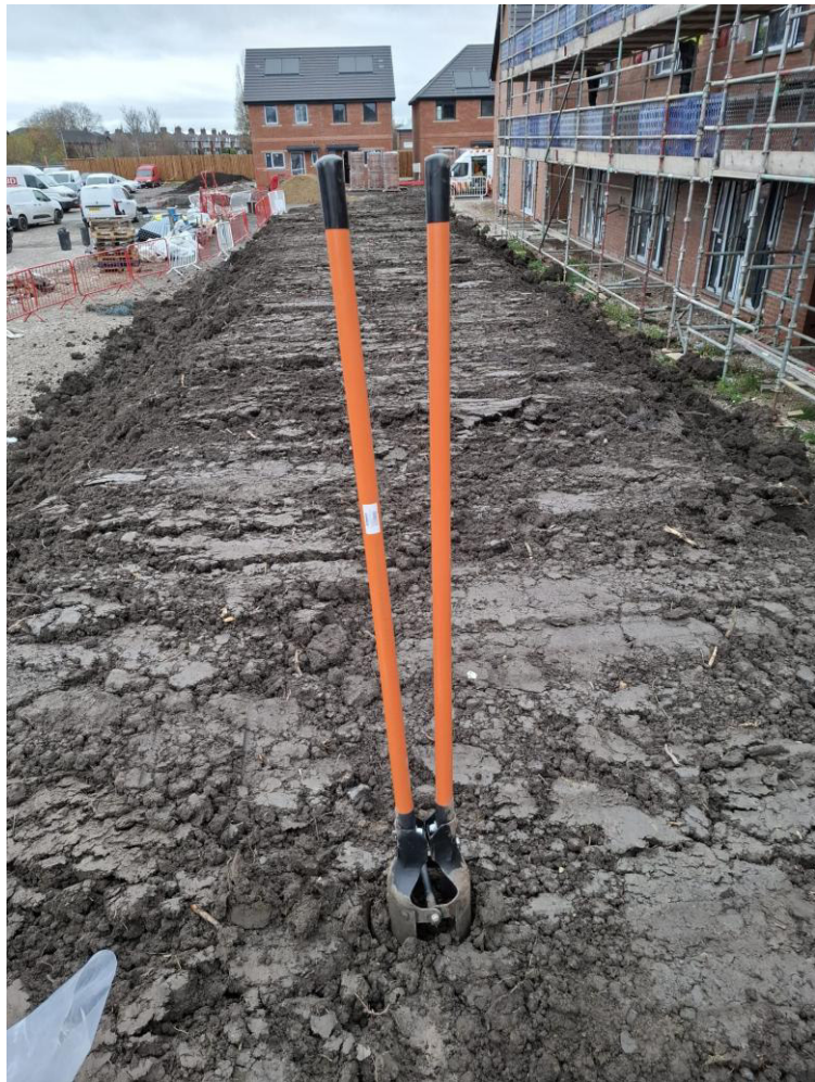
PHOTO 8: TS16-02 HOLE DIG VIEW
