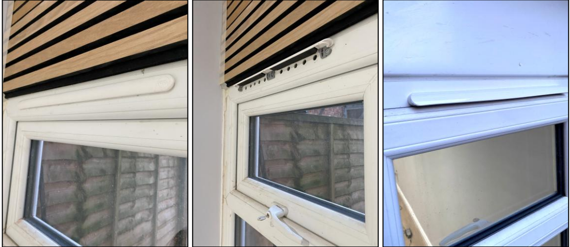
Figure 4.3 - Photographs showing frame-mounted sound attenuating trickle vent
