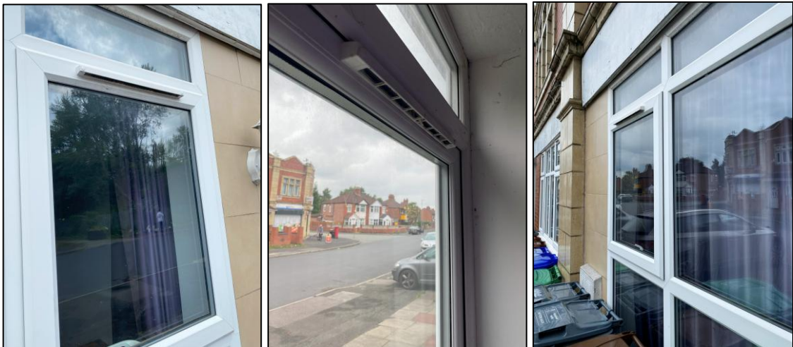
Figure 4.1 - Photographs showing double glazing and trickle vents to front elevation
