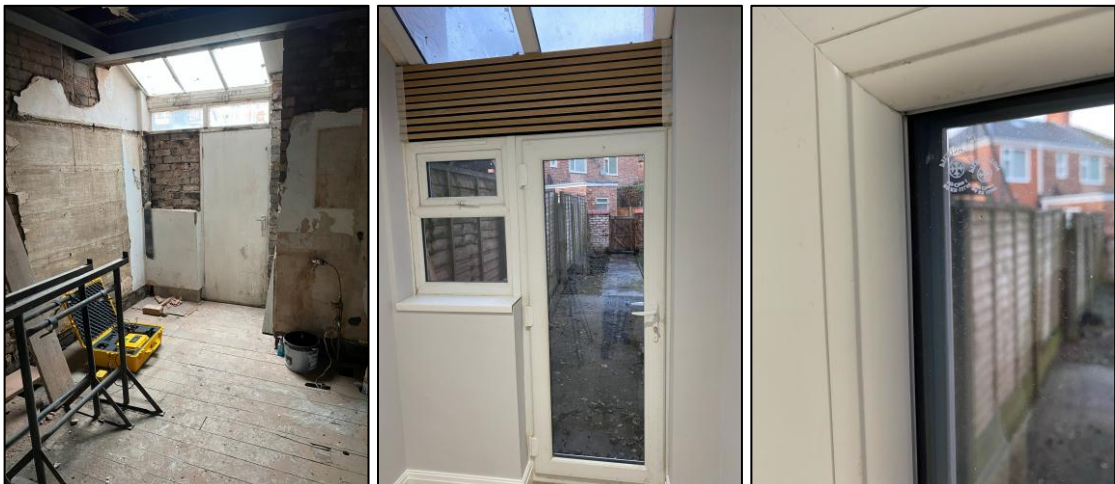
Figure 4.2 - Photographs showing previous rear door and new replacement door/glazing
