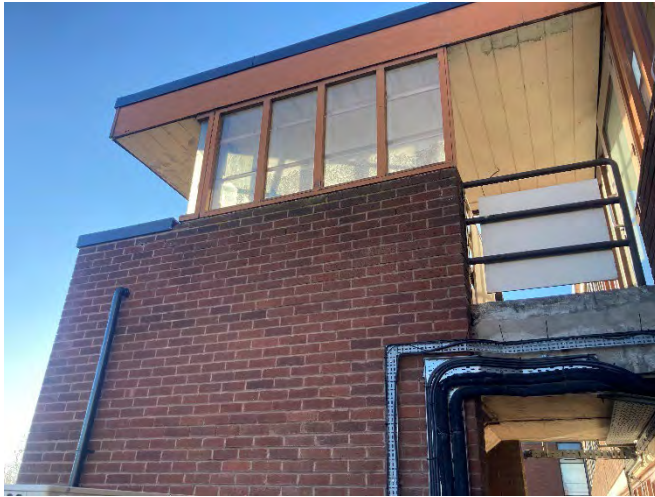
Photograph 4: Exterior of fire escape present on levels 4 and 5
