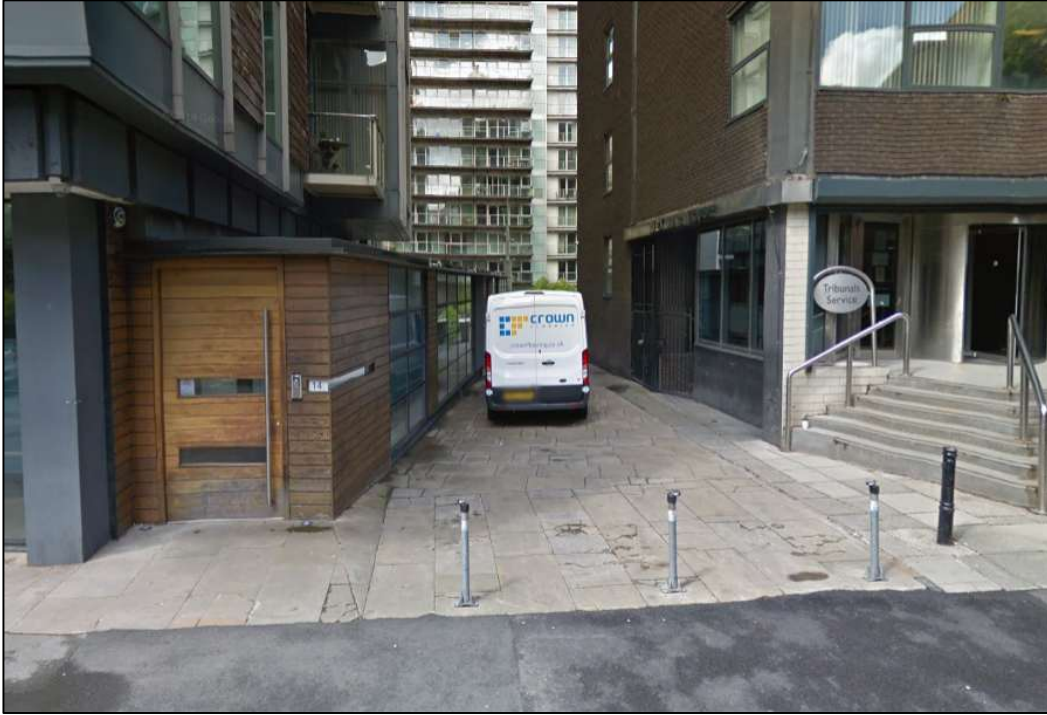
Figure 2: View of application site looking north towards the location of the proposed fencing and gates.
