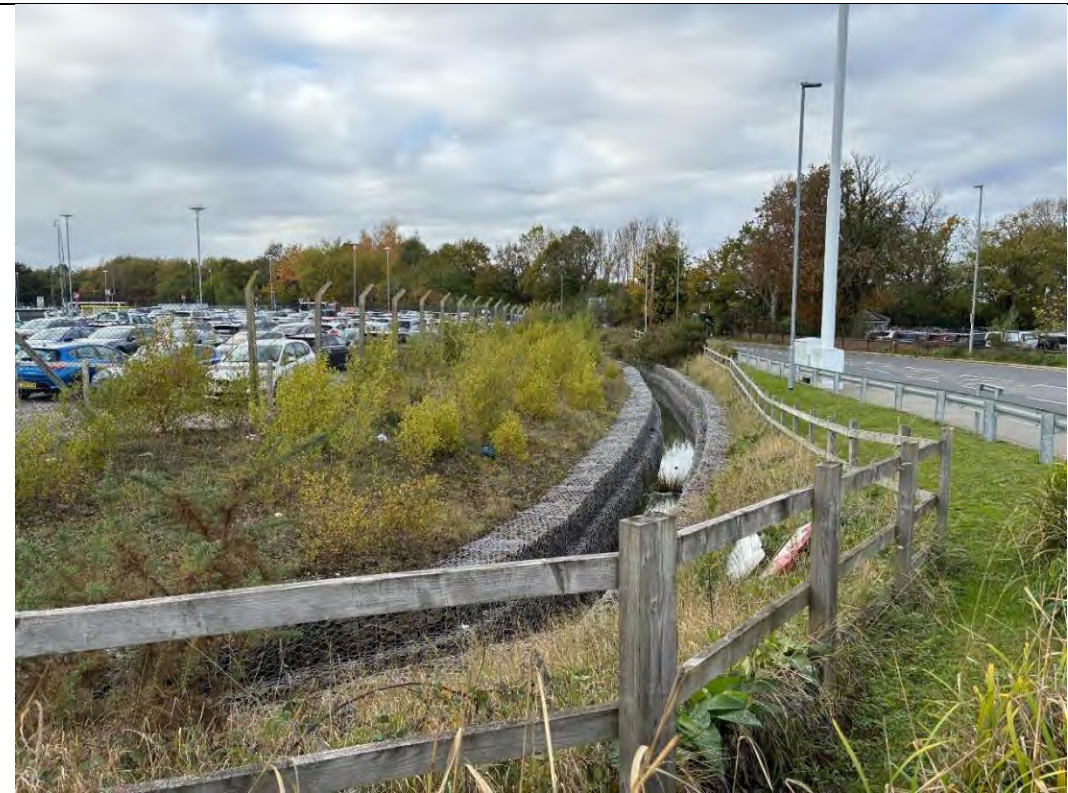
Plate 8: Drainage ditch running alongside Enterprise Way within the western part of the proposed development area.
