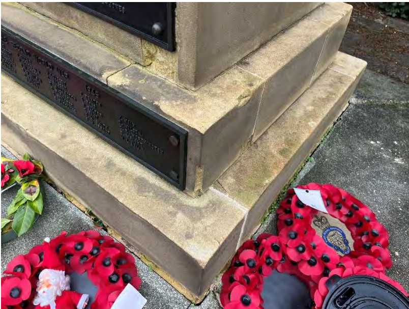
Photo 24 Right hand block, vertical vertex damaged to lower half
