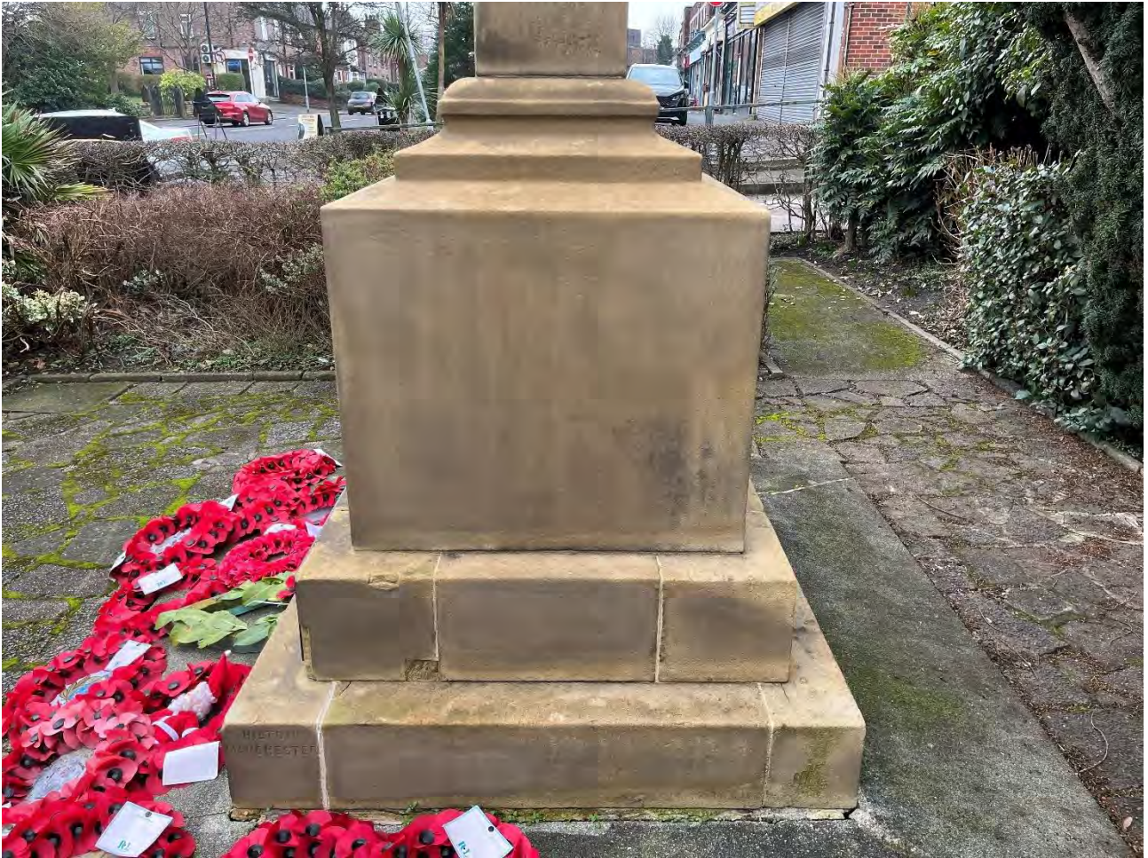
Photo 9 right elevation showing plinth and bases
