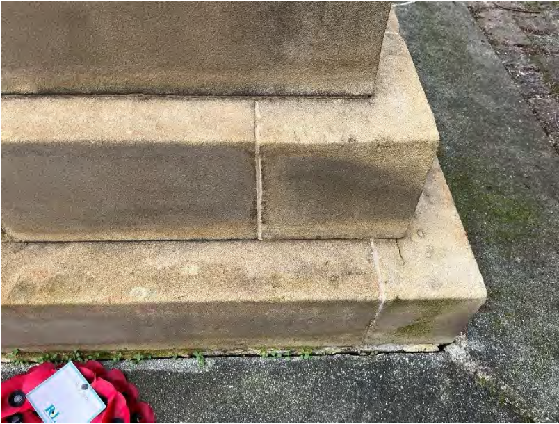
Photo 33 Rear joint re-pointed and slightly wider
