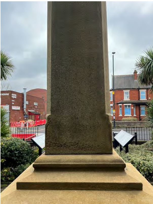
Photo 5 rear elevation showing lower shaft
