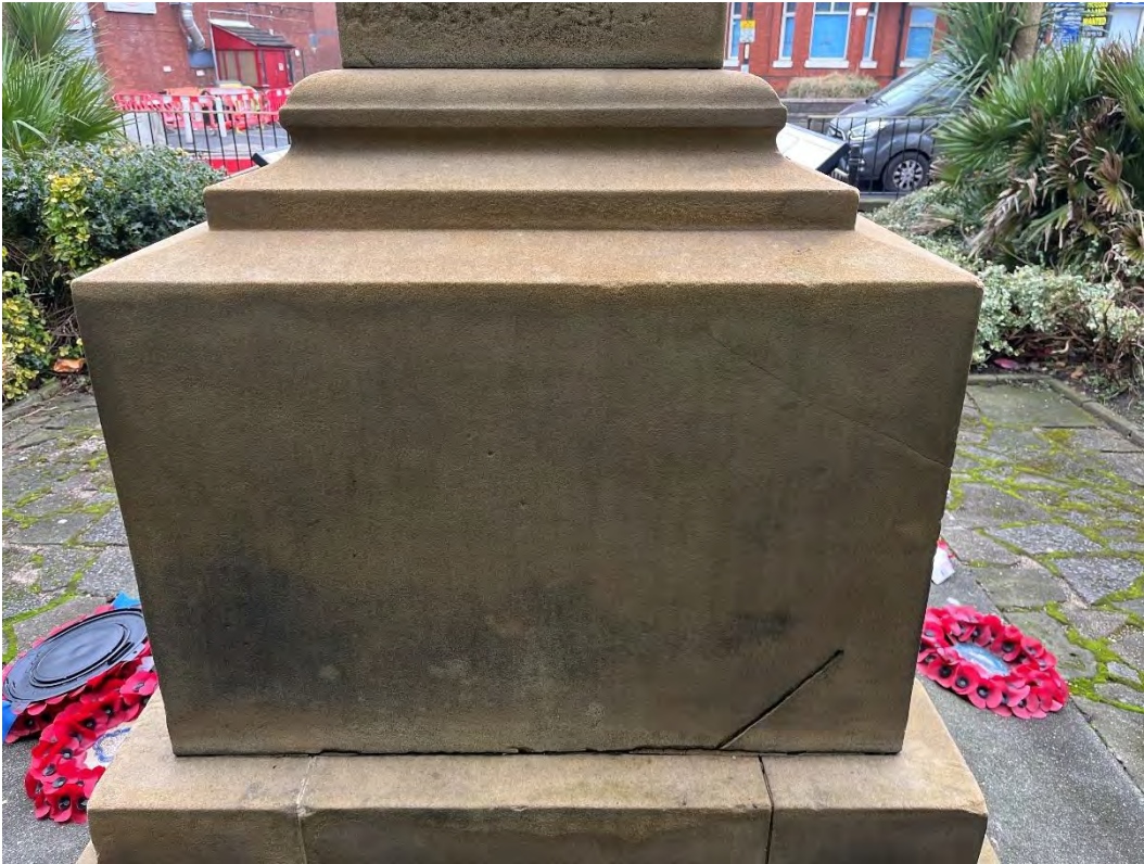
Photo 6 rear elevation showing plinth
