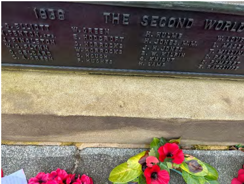
Photo 35 minor area of damage to upper surface in centre
