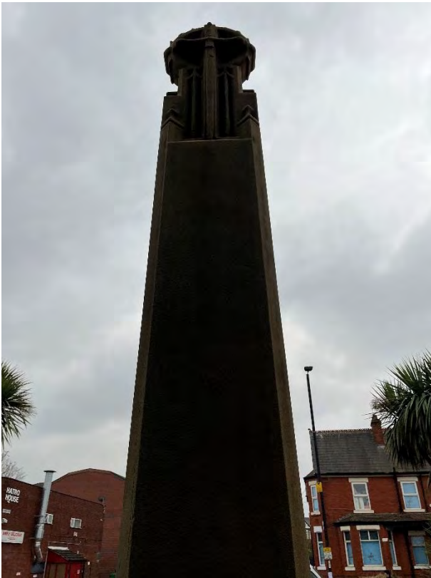
Photo 4 rear elevation showing upper shaft
