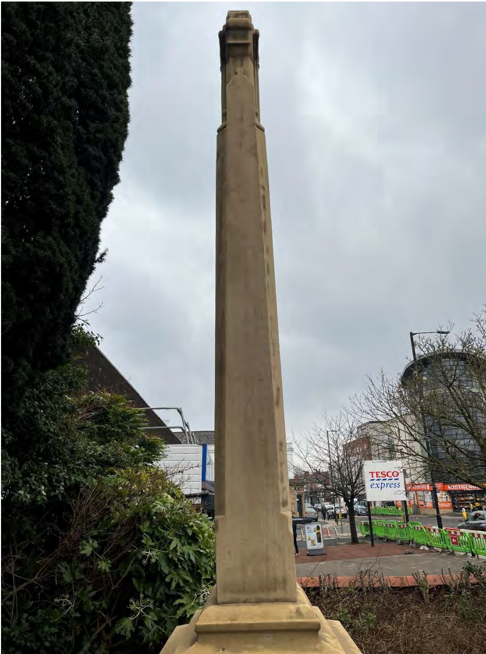
Photo 2 left elevation showing shaft
