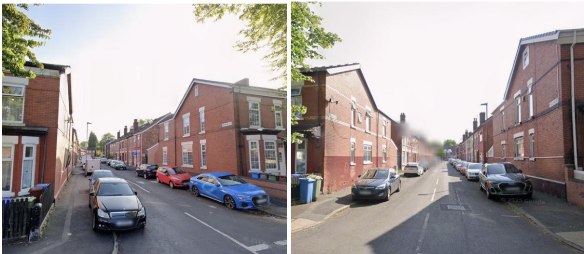
Figure 4: Properties in the area extending across their width of their plots (Left: Norburn Road – Right: Palm Street)
