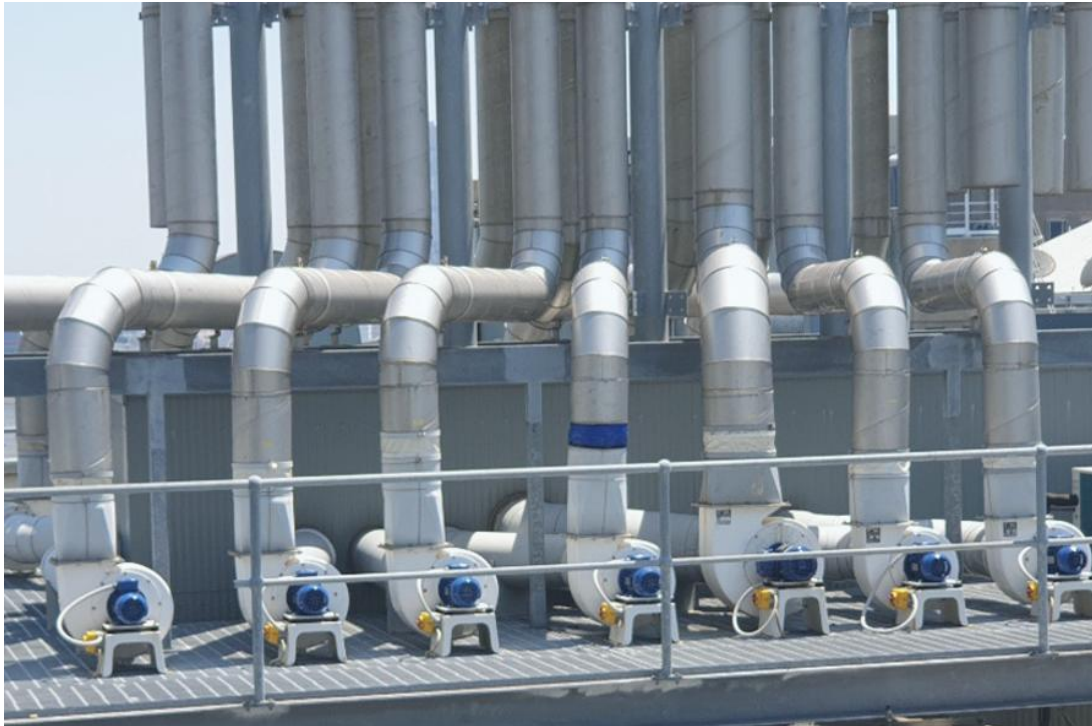
Figure 3 – Typical Fan Arrangement at roof level
