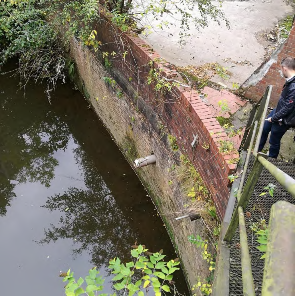
Figure 5-1 Existing Outfall Observed During Site Visit
