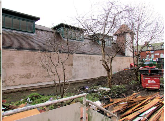
View South Towards Site
