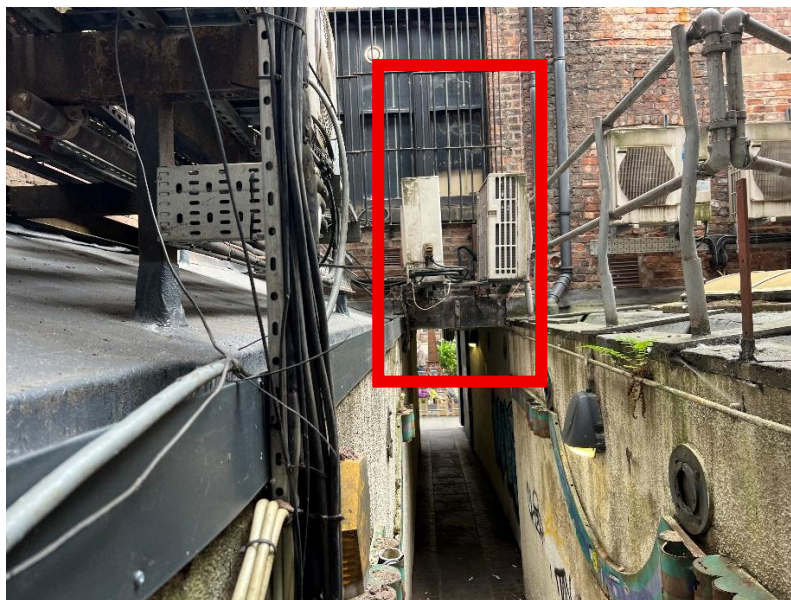
Figure 3 - Overview of rear elevation and adjacent plant
