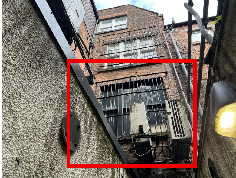
Figure 2 - Image of rear elevation and existing condensers
