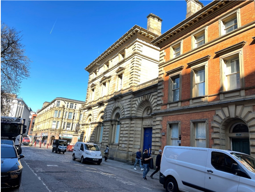
Figure 1 - Photograph of 25 St Anns Street from St Anns Street
