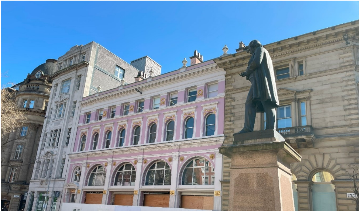
Figure 2 - Photograph of 17 St Anns Square from St Anns Square
