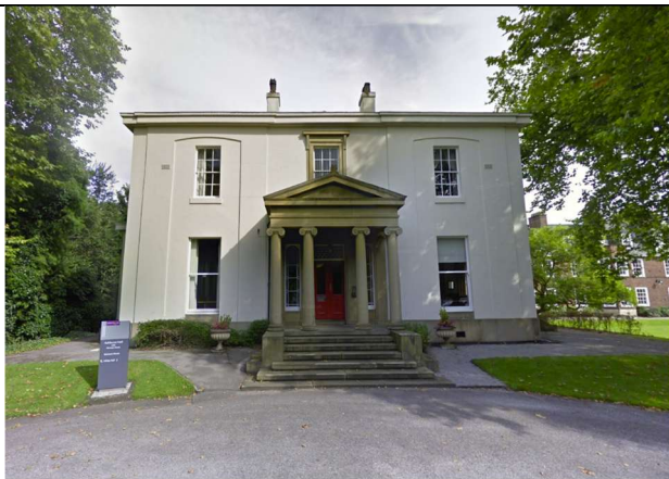
Image 5 – Behrens Hall – South facing elevation
