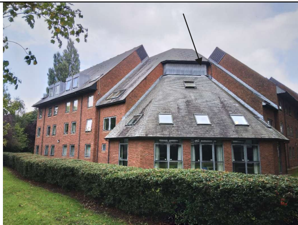
Image 1: Sheavyn House - Southwest facing elevation
