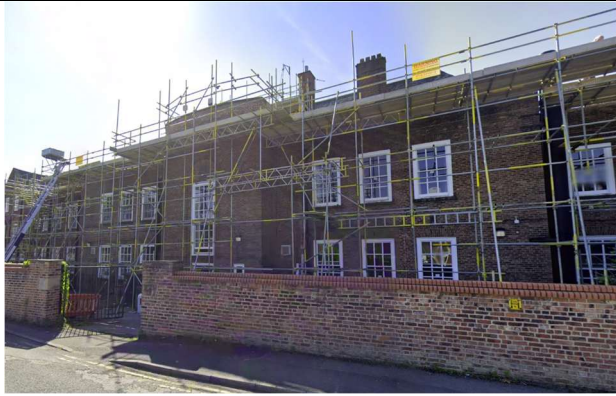
Image 3: Ashburne Hall – East facing elevation
