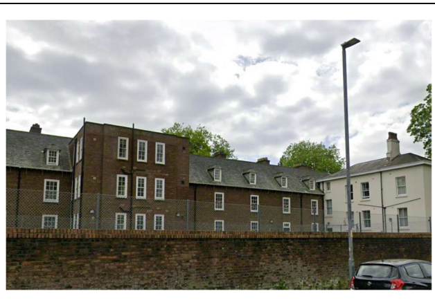
Image 6 – Behrens Hall – North facing elevation
