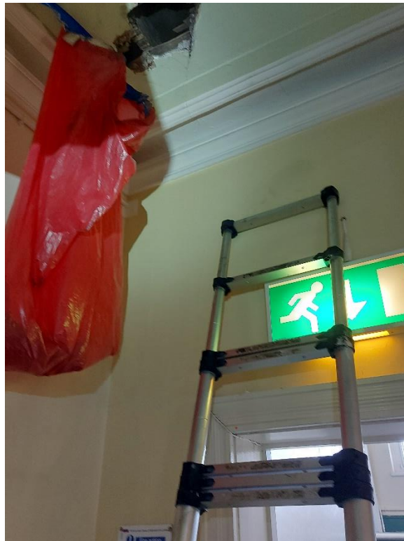
Photograph 8 Landing 1.C03 – ceiling joists exposed
