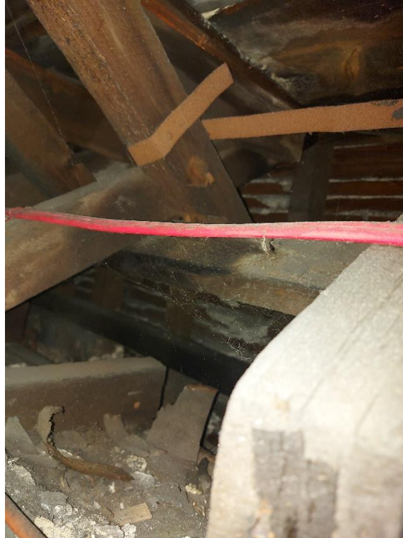
Photograph 5 Room 1.107 – rafter and hip feet appear intact
