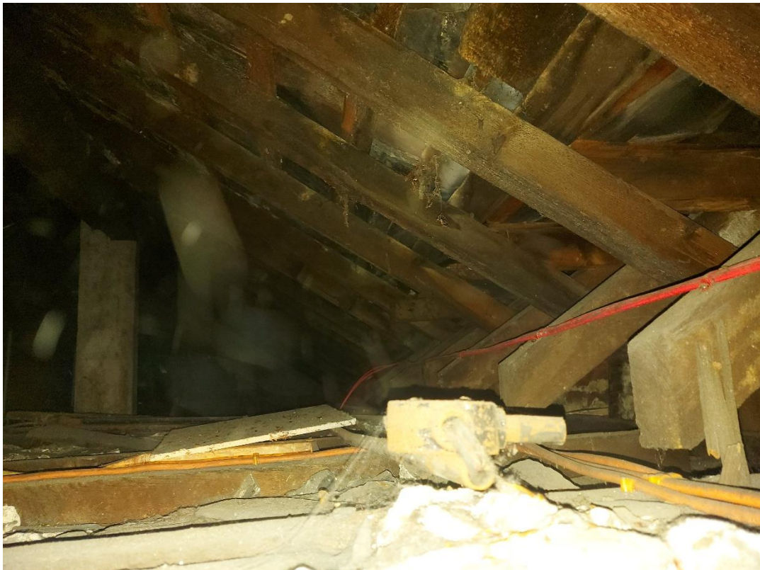
Photograph 4 Room 1.107 – rafter feet appear intact
