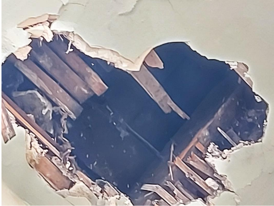
Photograph 7 Stairway 1.024 – rafter feet appear intact
