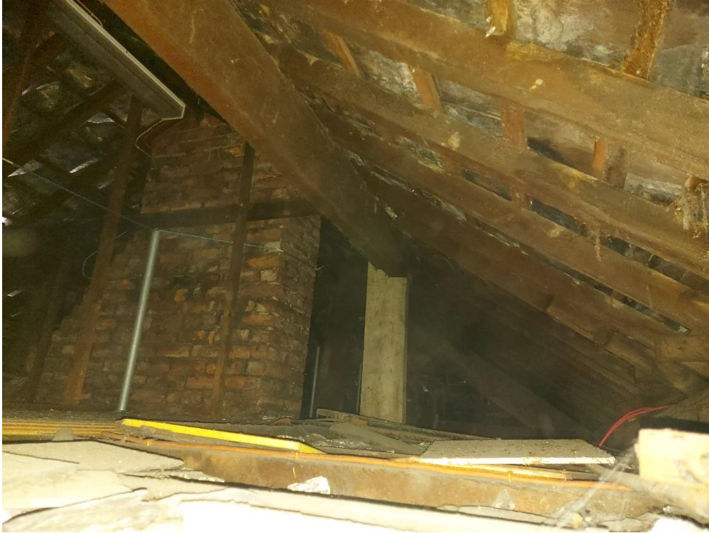
Photograph 3 Room 1.107 – main roof carcass appears intact
