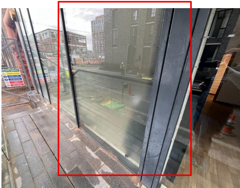
Glazed window to be replaced with door on Ellesmere Street
