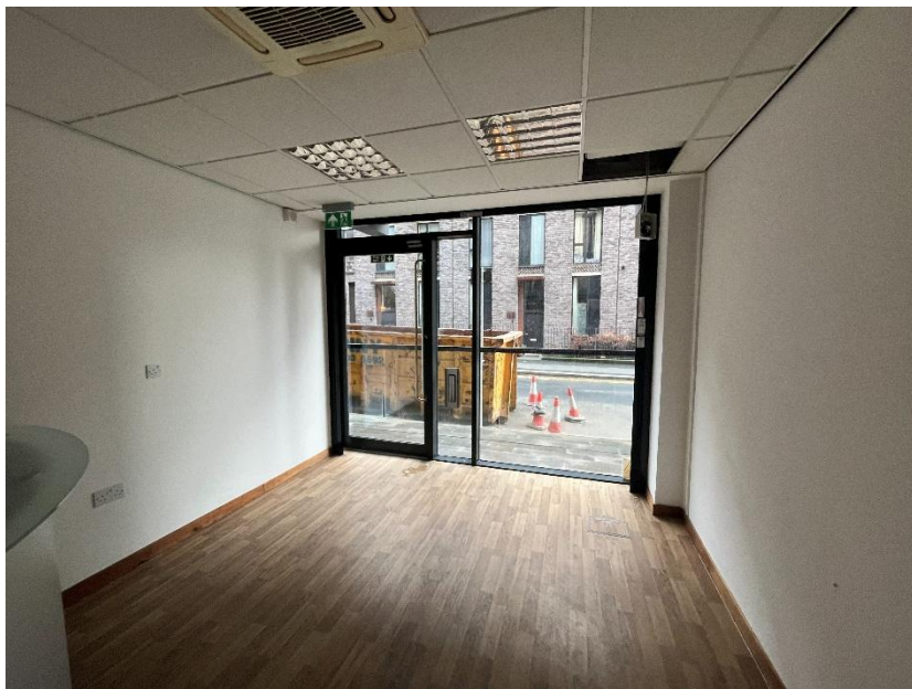
Existing internal view off commercial space with door and window screen
