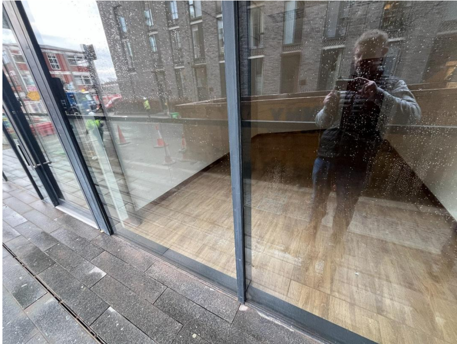
External pavings level with windows and doors on Ellesmere Street
