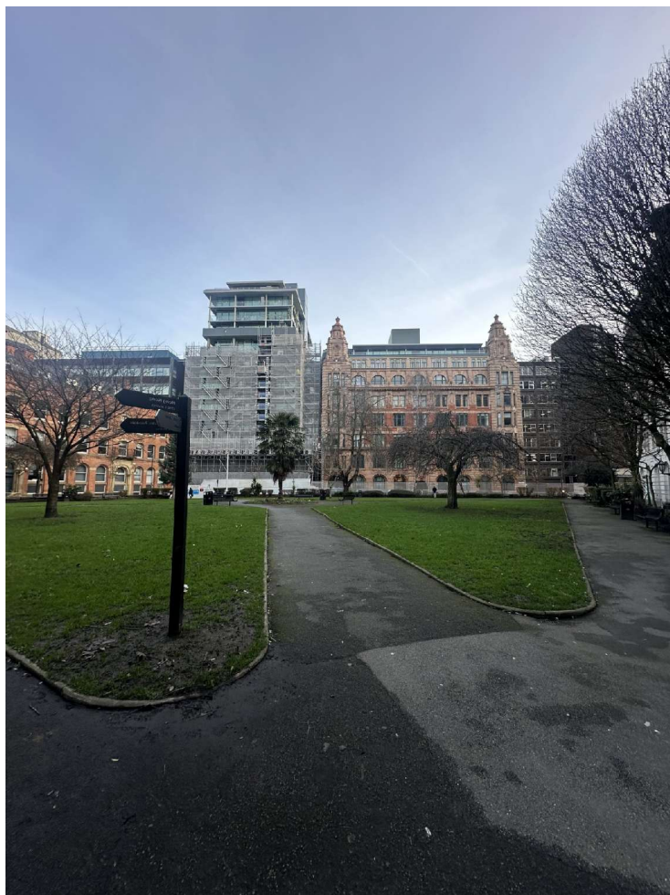
View of Century Buildings and Alexandra House from Parsonage Gardens.
