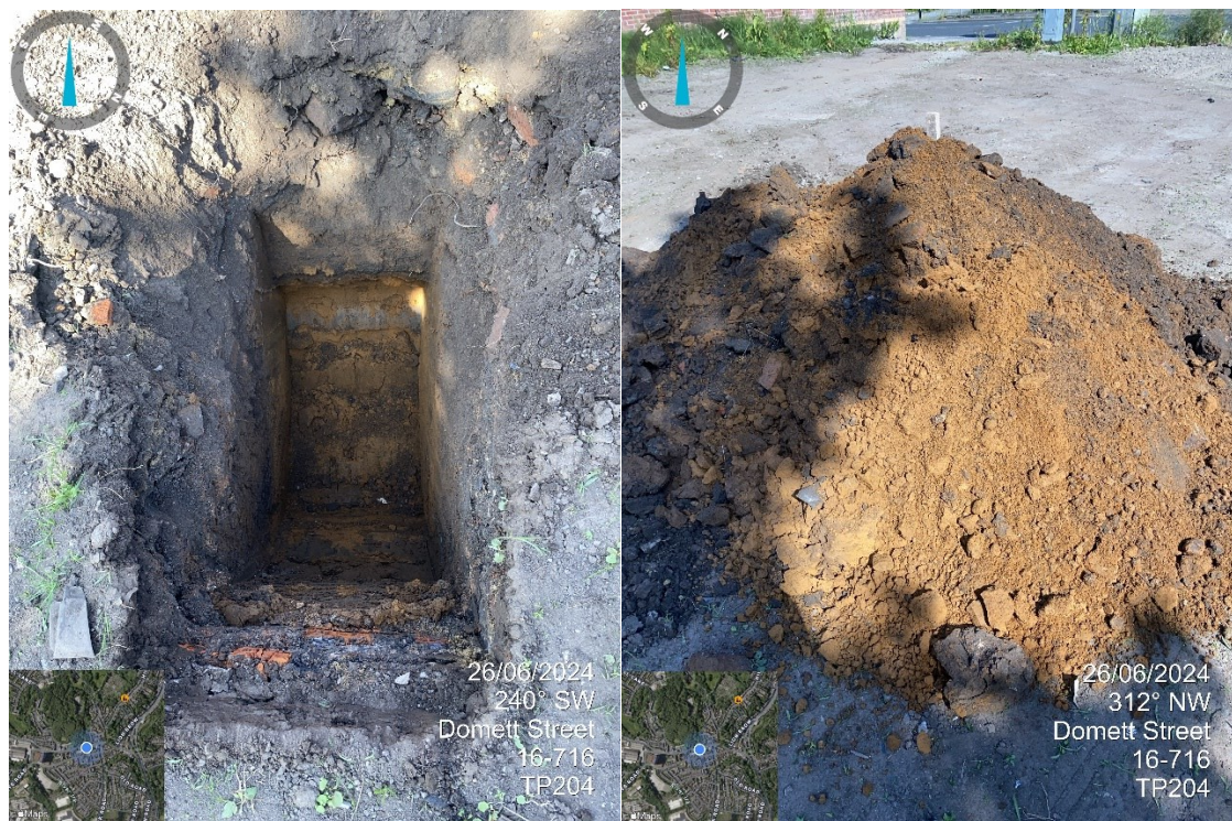
PLATE 6 TP204 PIT AND ARISINGS
