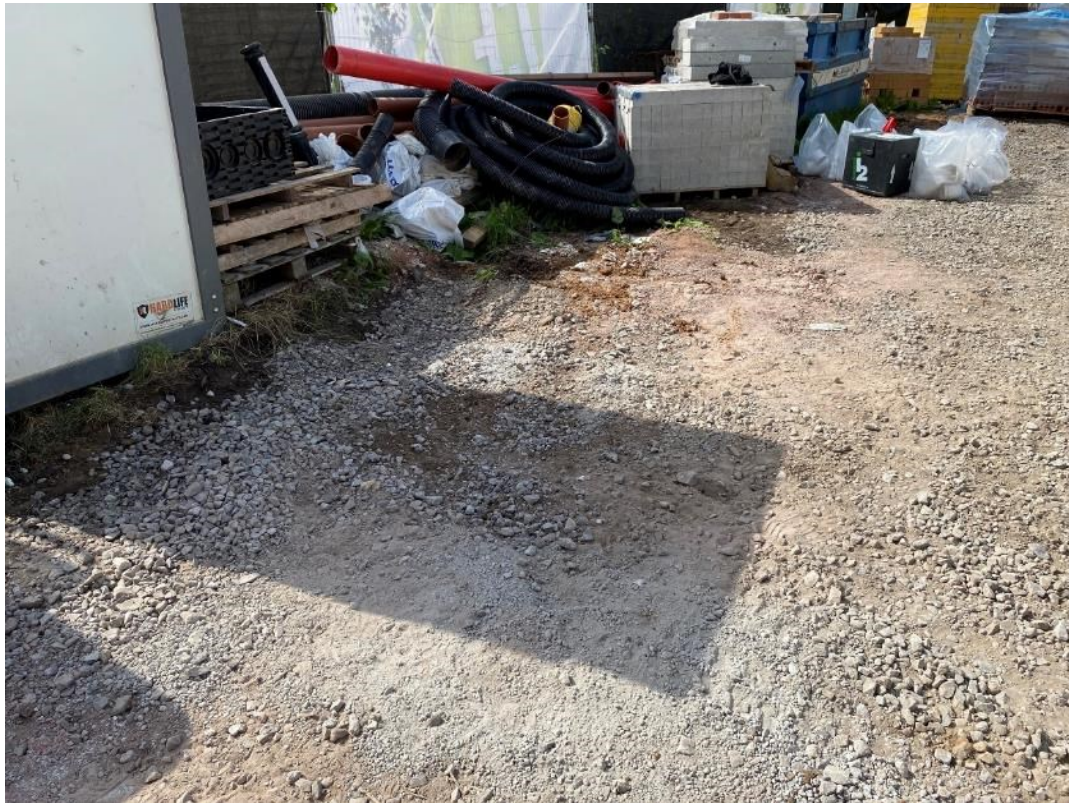
PLATE 1 STORAGE OF CONSTRUCTION MATERIALS
