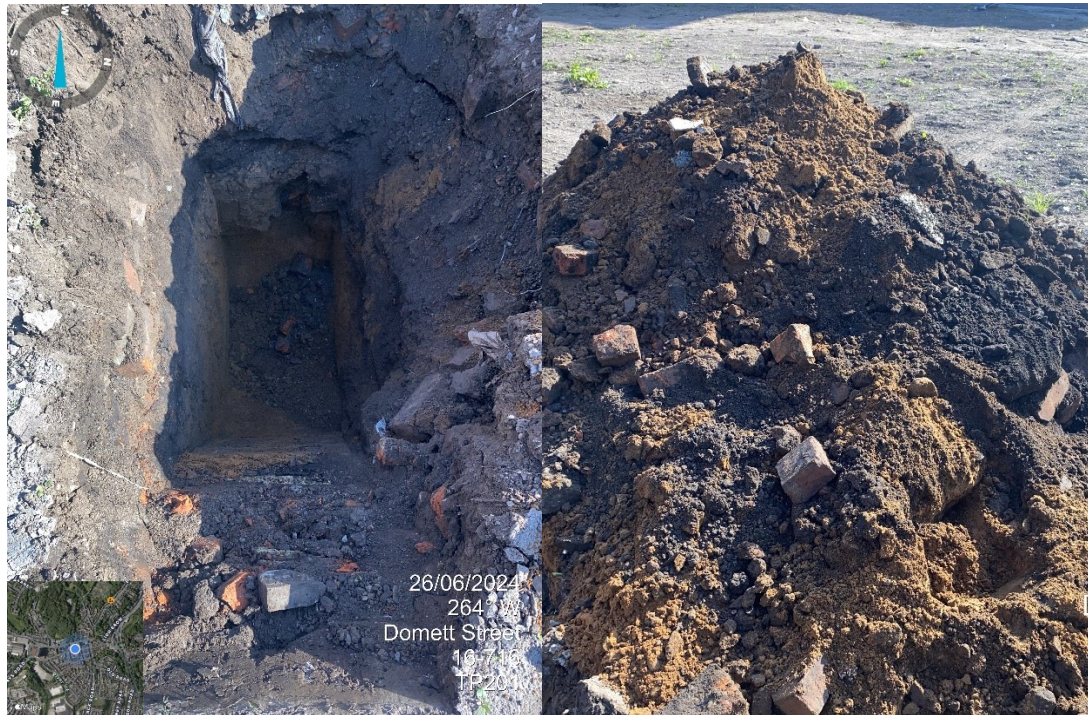
PLATE 5 TP201 PIT AND ARISINGS
