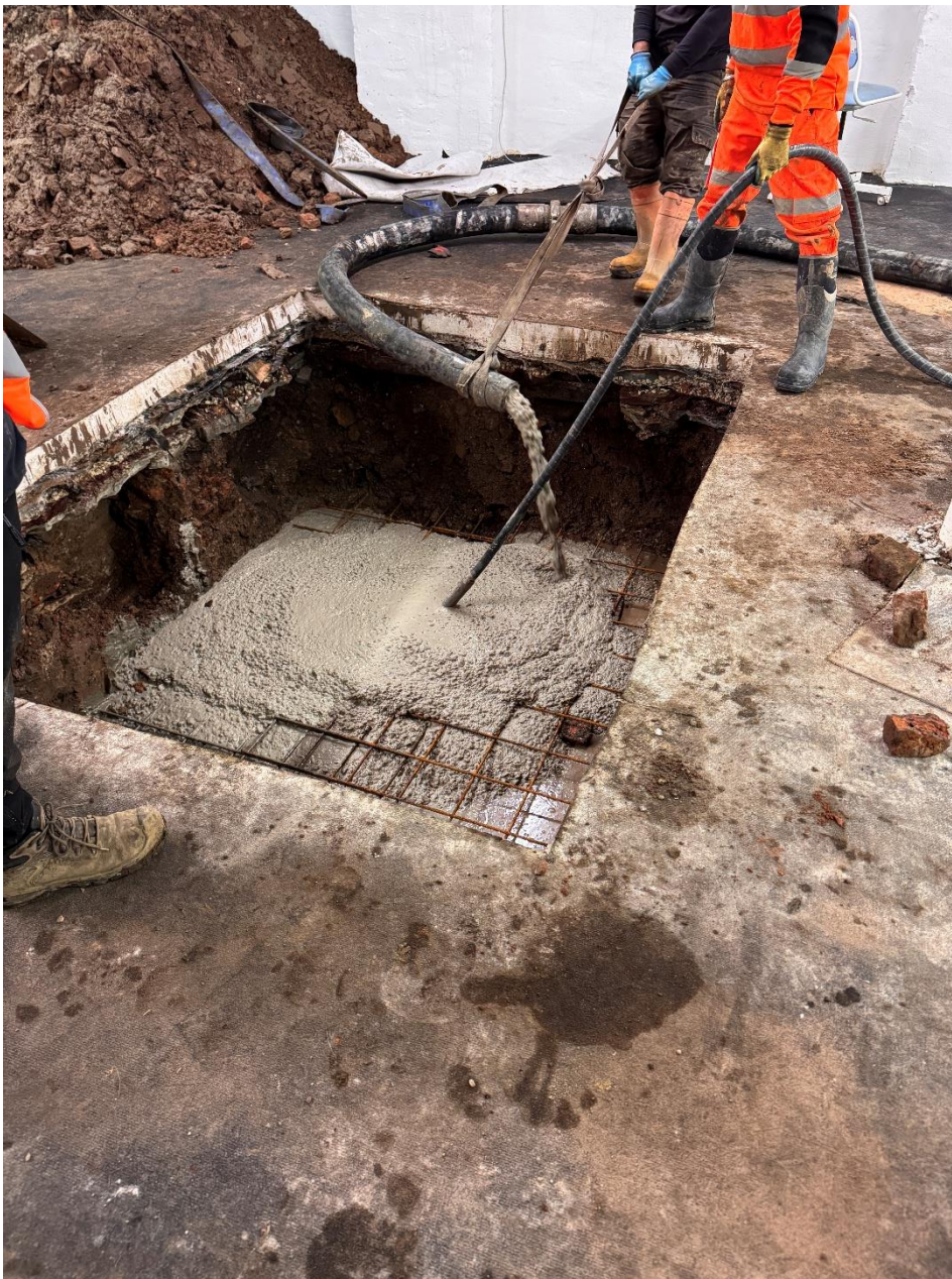
Enclosure 1: Photographic evidence of Material Operation comprising the commencement of the construction of an internal supporting column.
