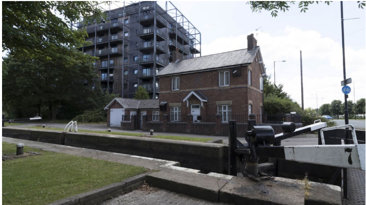
Ashton Canal Lock Keeps Cottage and Lock no7
