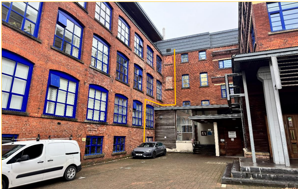
Photograph 1 East Elevation (proposed pipe route marked in yellow)
