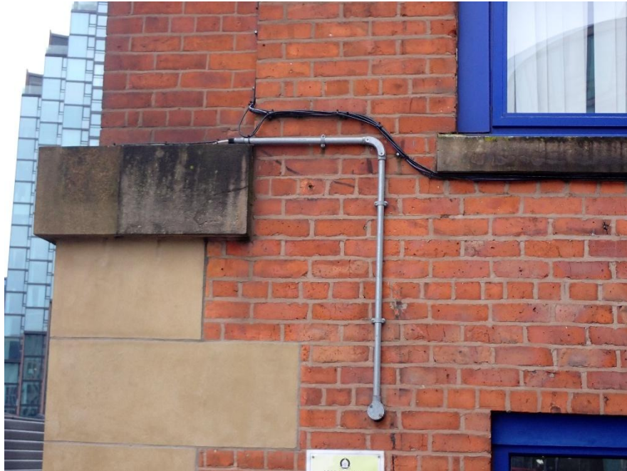
Photograph 2 Typical Surface Fixed Services
