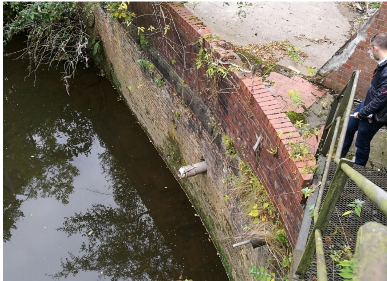
Figure 5-1 Existing Outfall Observed During Site Visit
