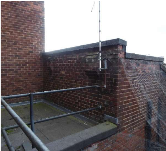
Stage right Fly Tower wall
