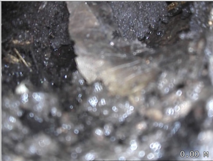
Start node type, manhole, reference MH01
