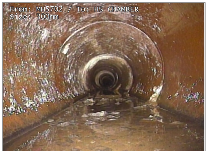
Survey abandoned - Remark: UNABLE TO PASS DEBRIS CLEANSE REQUIRED
