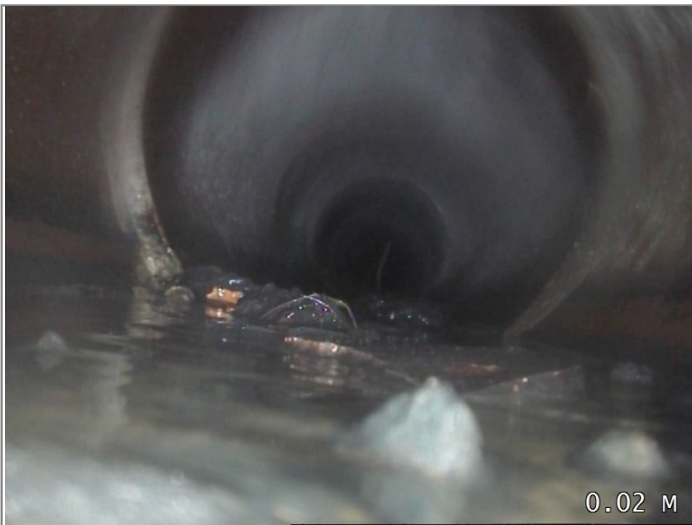
Start node type, manhole, reference MH5702
