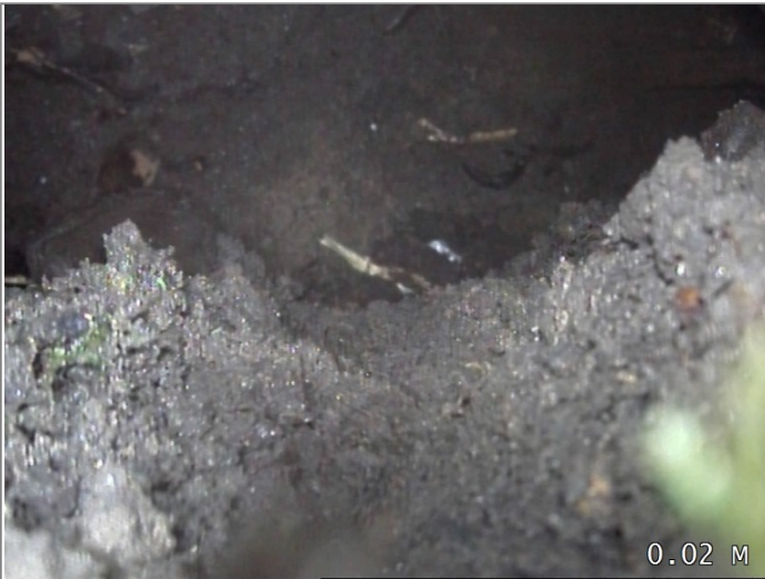
Start node type, manhole, reference MH01
