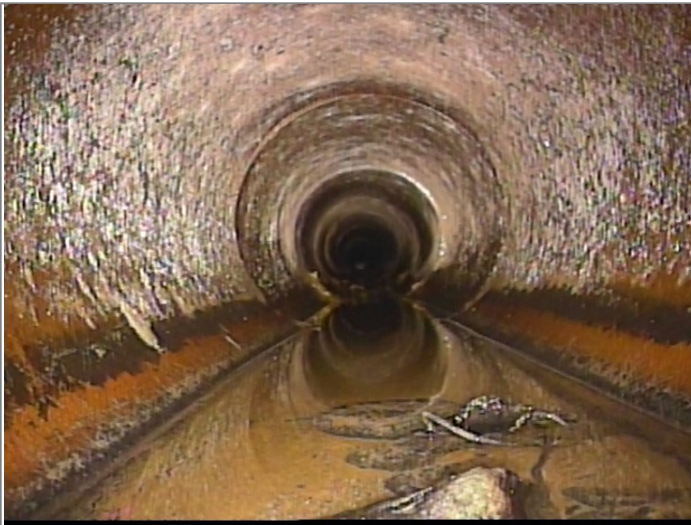
Start node type, manhole, reference MH5702
