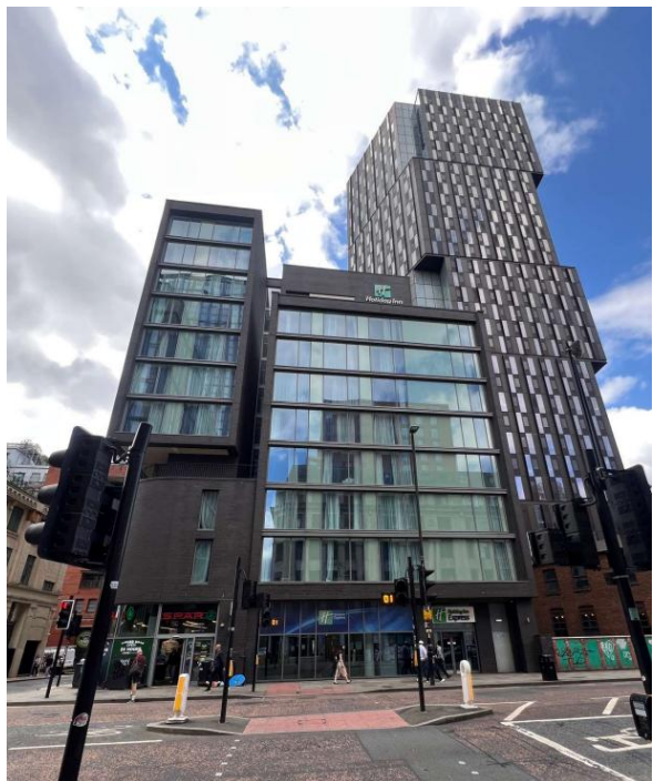
Figure 1 – Existing Oxford Road elevation
