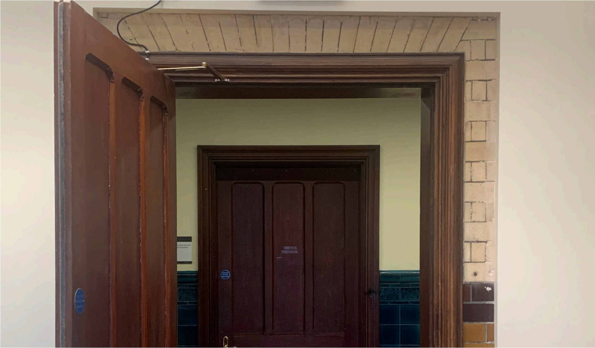
▲ Insulated Plasterboard Lining to be Removed if safe to do so to Reveal Historic Brickwork
