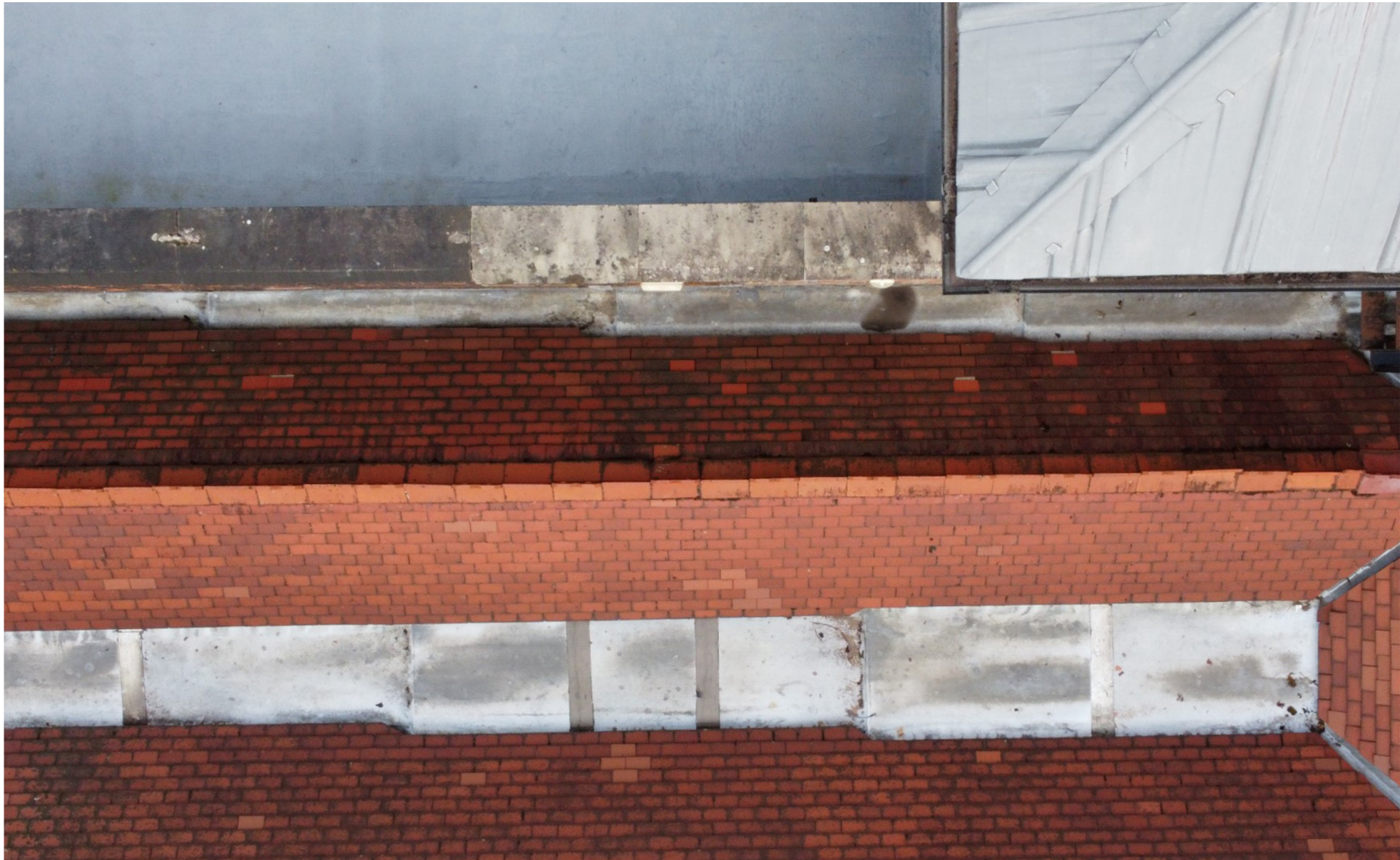
▲ View of Roof from Drone
