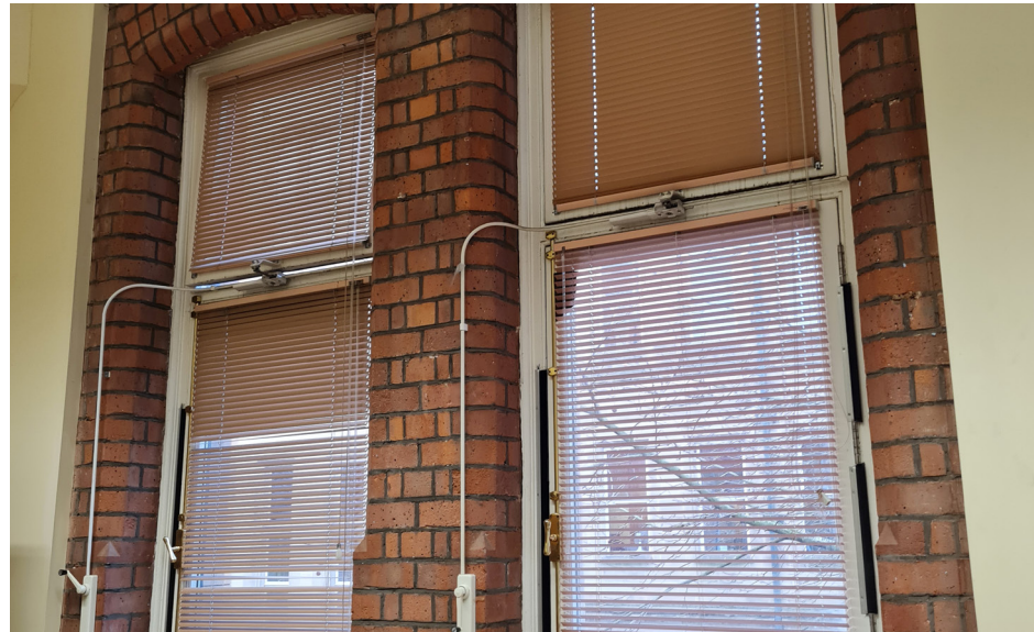
▲ Surface mounted dado trunking, containment and services within cellular spaces
