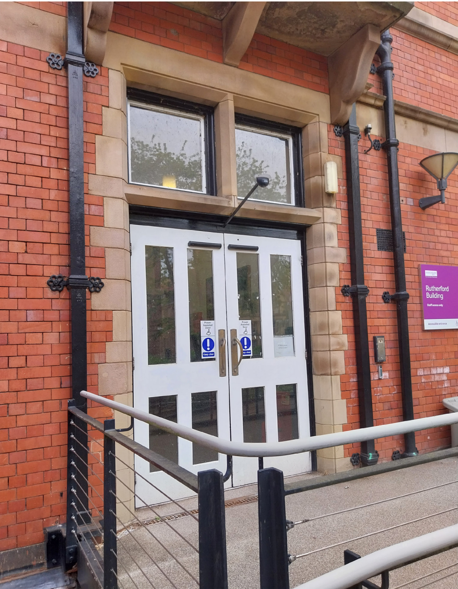
▲ Replacement of Entrance Doors to West Elevation
