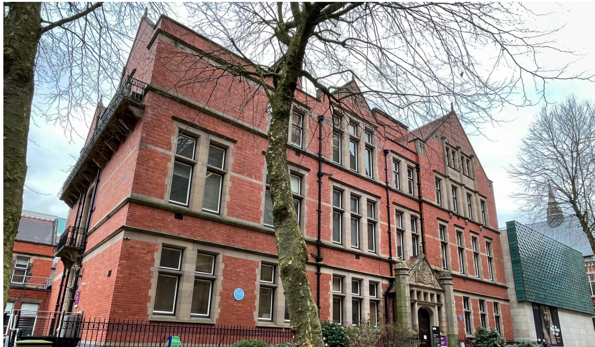
▲ Coupland Street External Facade
