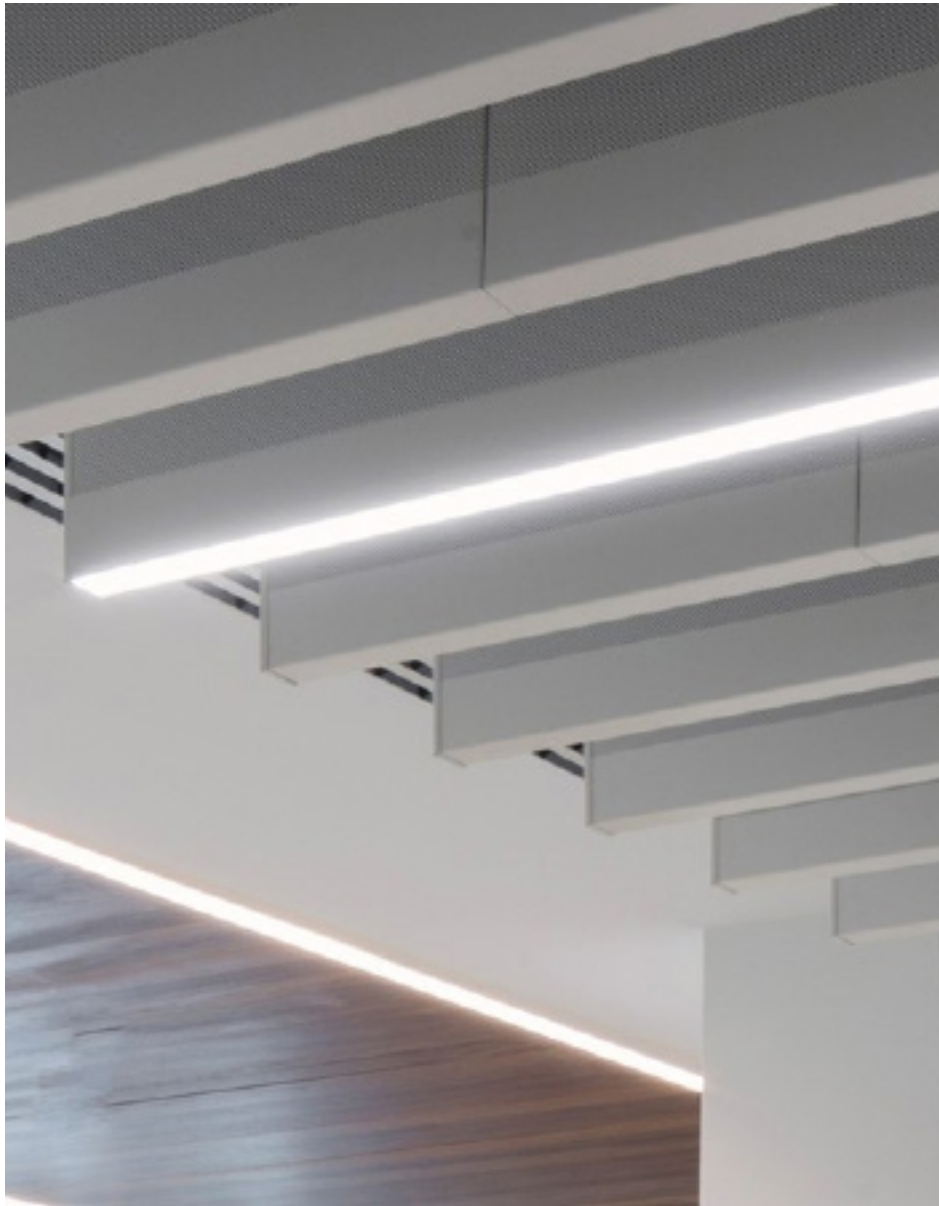
▲ Integrated Lighting with Linear Acoustic Baffles
