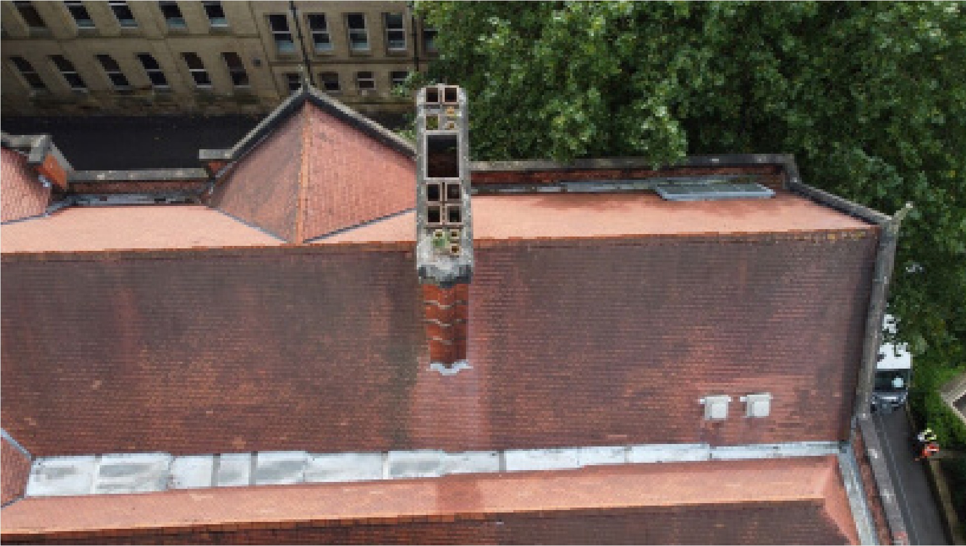
▲ Existing Lead Gutter over Corridor
