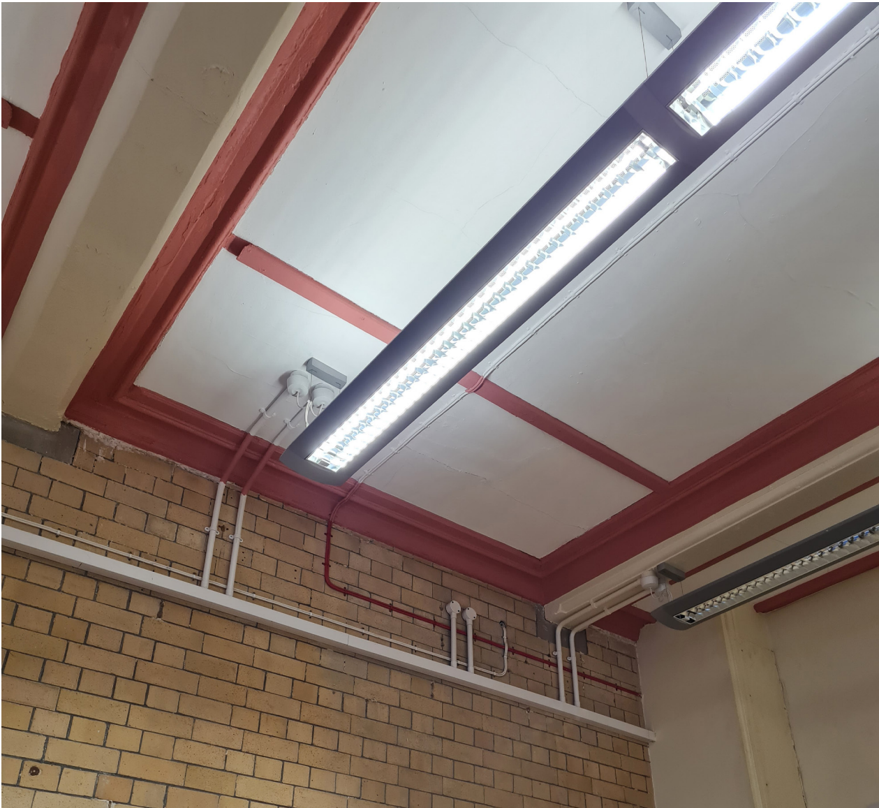
▲ Existing Cornices to be Retained wherever Possible and Reinstated like-for-like, where Removal due to Remediation is Required
