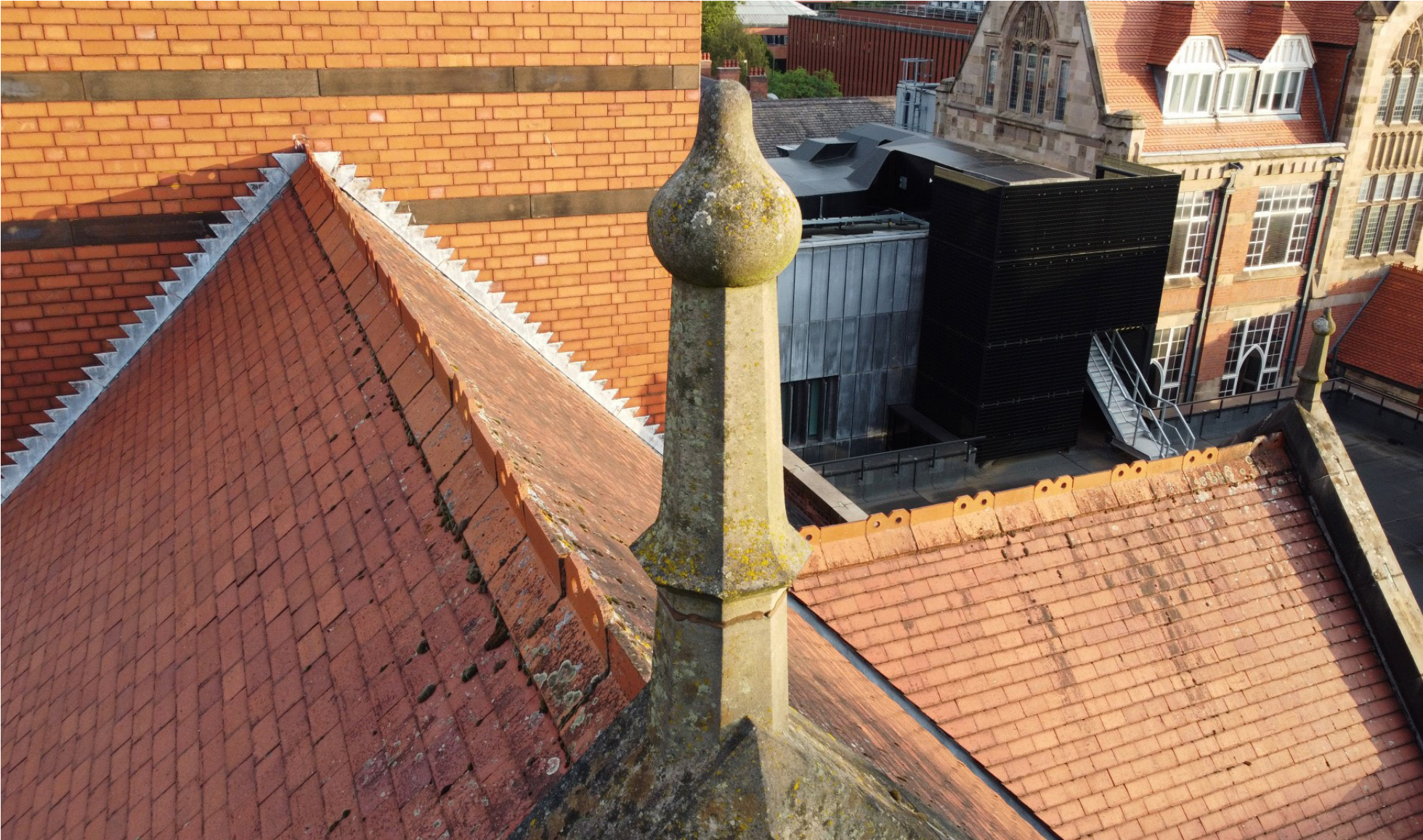
▲ View of Roof from Drone
