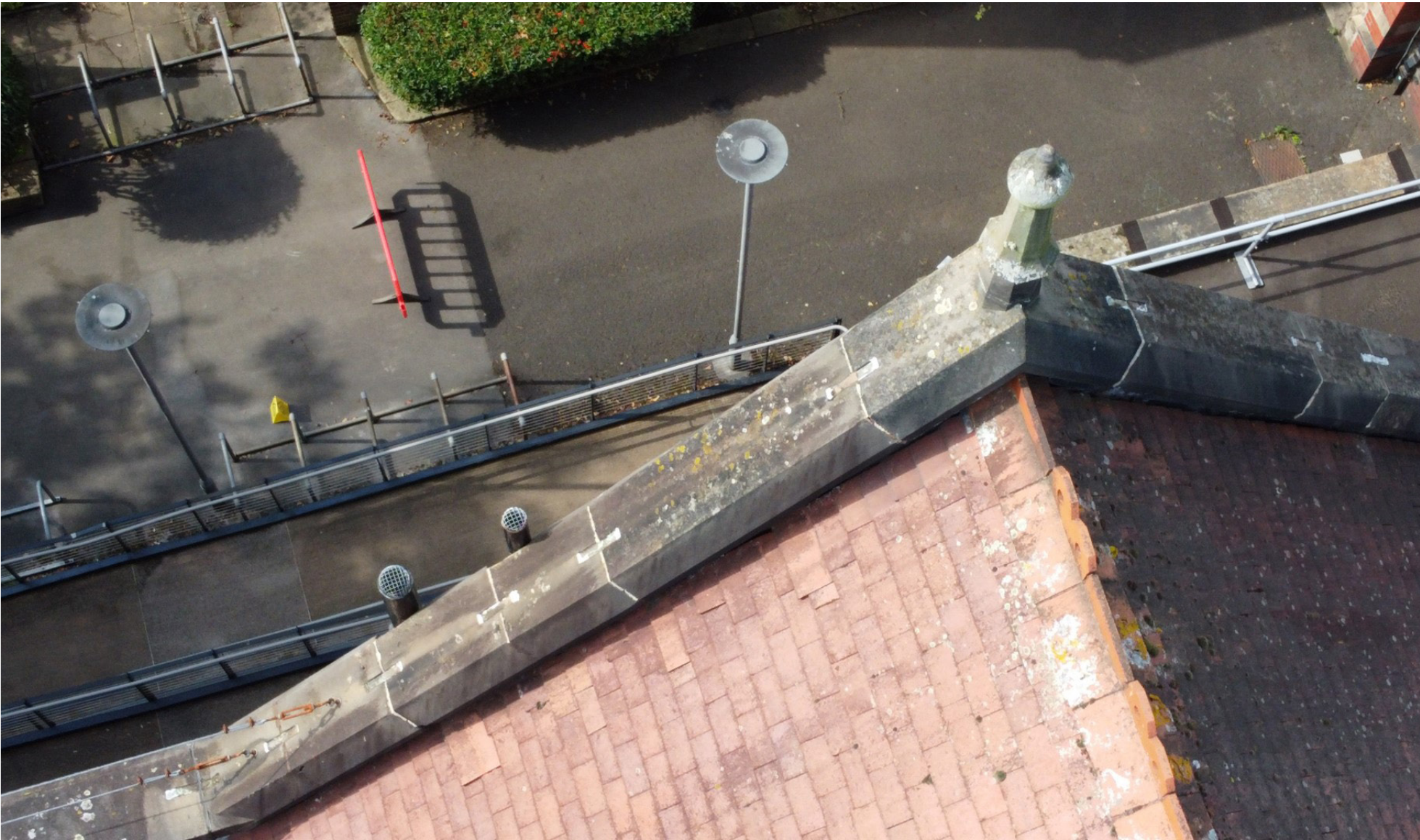
▲ View of Roof
