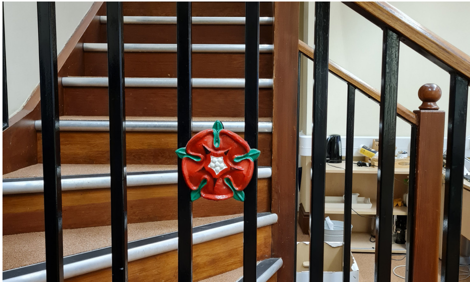
▲ Late addition - balustrade to mezzanine floor
