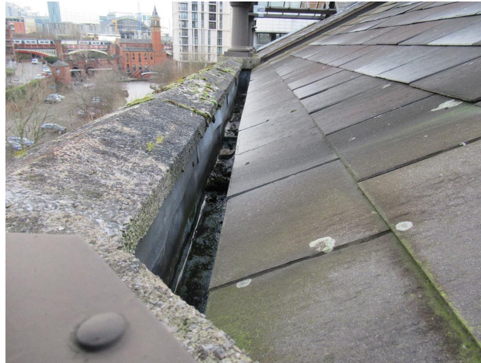
2. Lead lined back parapet gutter
