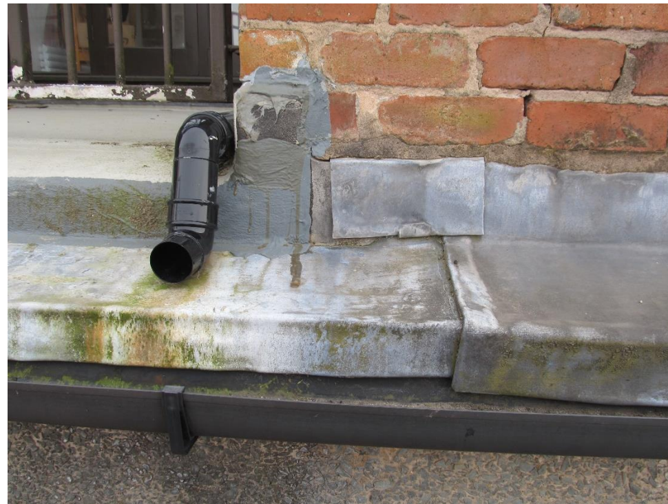
2. Lead lined back parapet gutter
