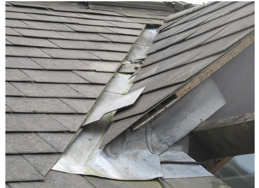
3. Lead lined back parapet gutter
