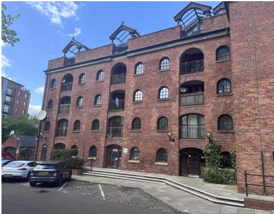
10. General view of the LHS elevation
