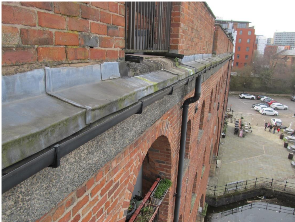
4. Eaves guttering and downpipe
