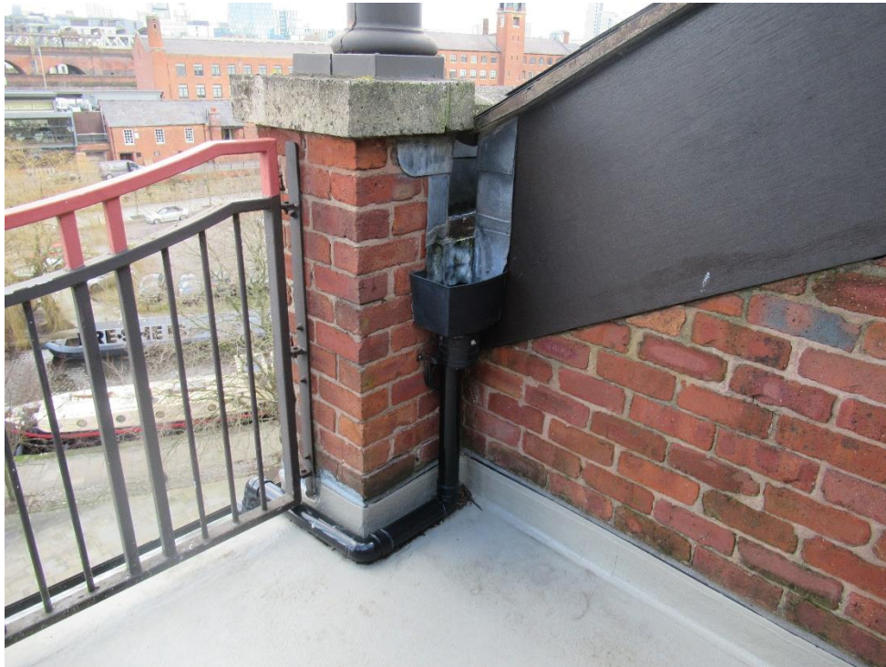
1. Back parapet gutter draining to hopper and downpipe that runs into eaves guttering
