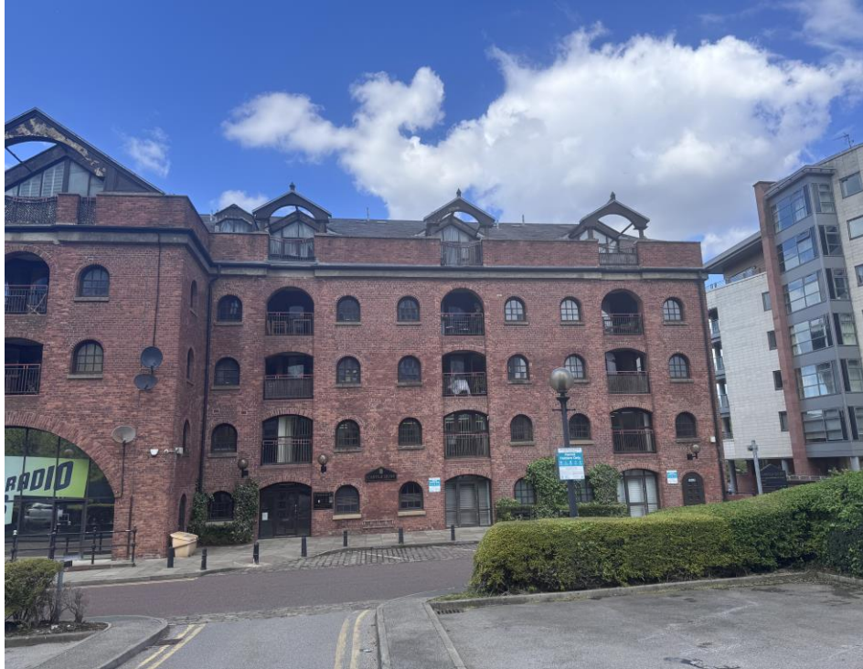
7. General view of the RHS elevation
