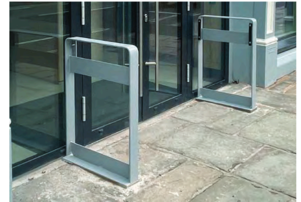
Existing door guarding
