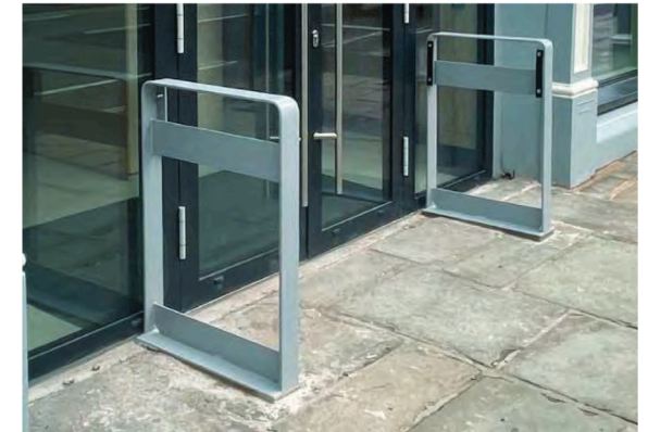
Existing door guarding
