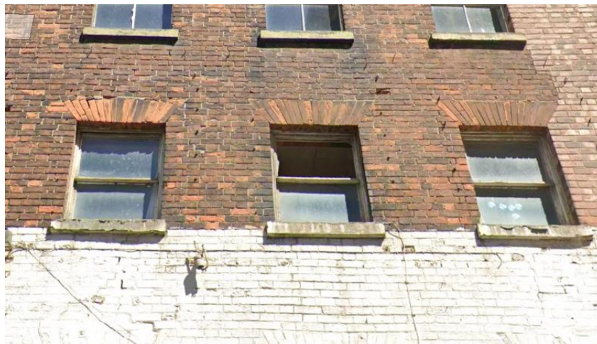
Photo showing embedded metalwork within elevation (small black shadows on regular grid between windows)
