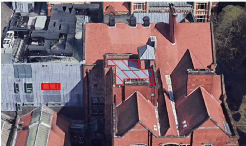
Figure 7 Mark-up of worst affected window in relation to rooftop plant location
