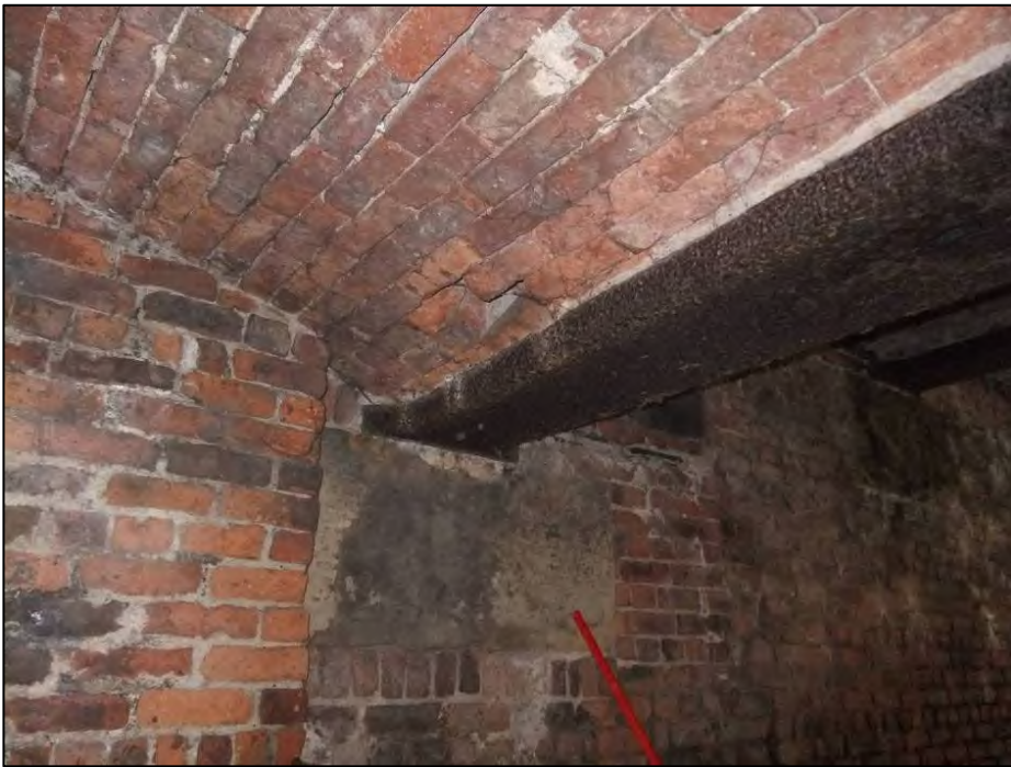
Plate 5 Culvert B24 wall of mixed materials
