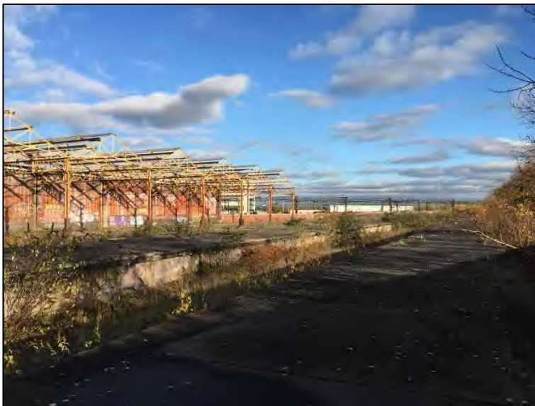
Plate 2 - Western section of the former railway station platform, looking east
