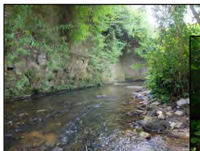
Looking downstream from culvert
