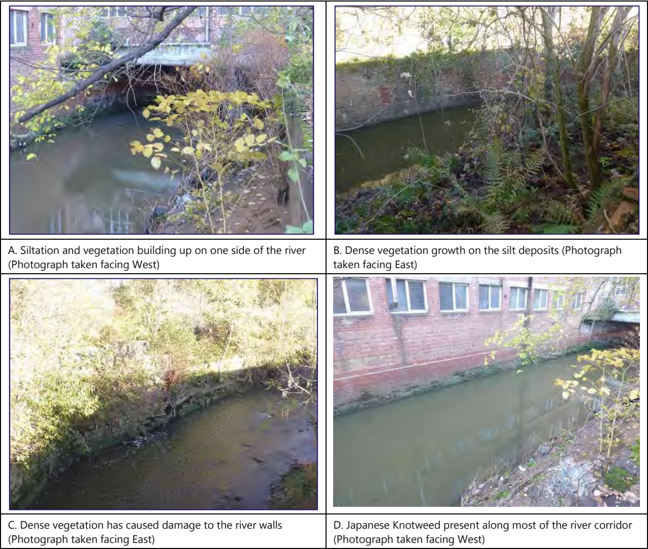
Figure 3-1 Site visit photographs
