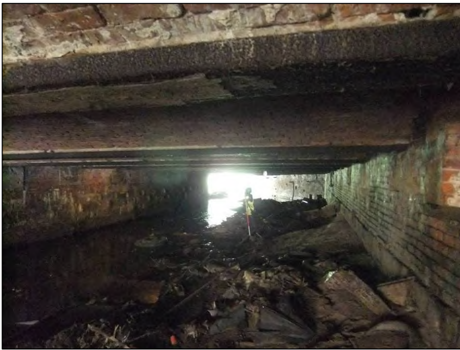
Plate 3 Culvert B24 box section culvert over River Medlock
