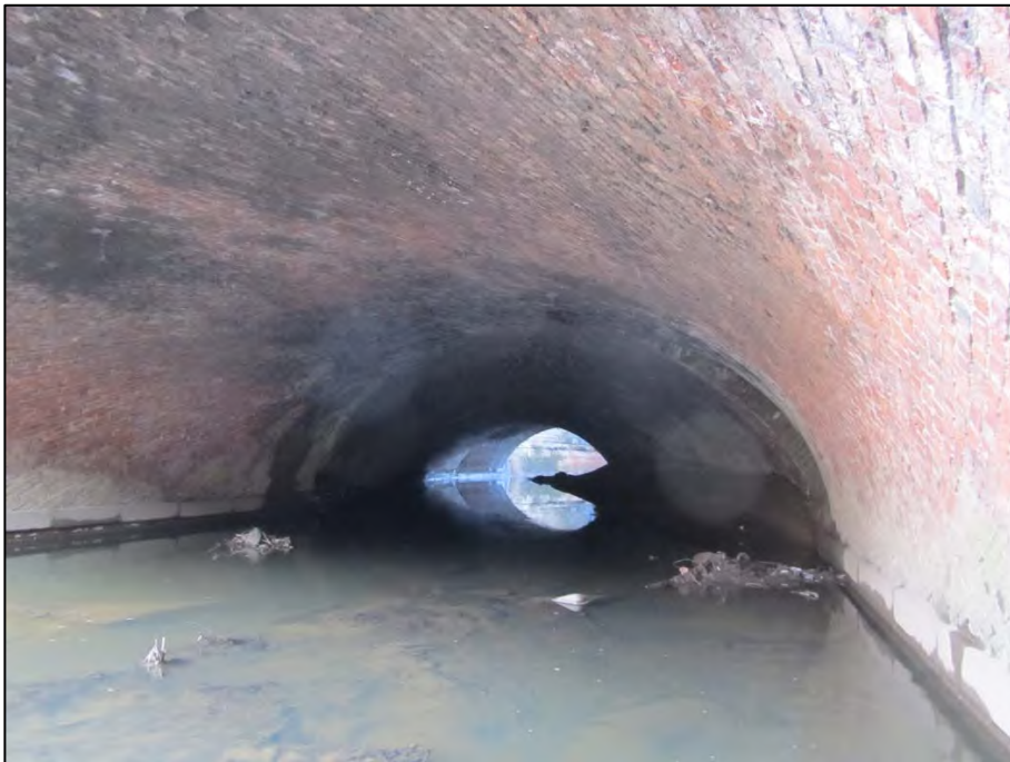
Plate 8 Culvert B26 looking upstream, showing intact brickwork interior (February 2019)
