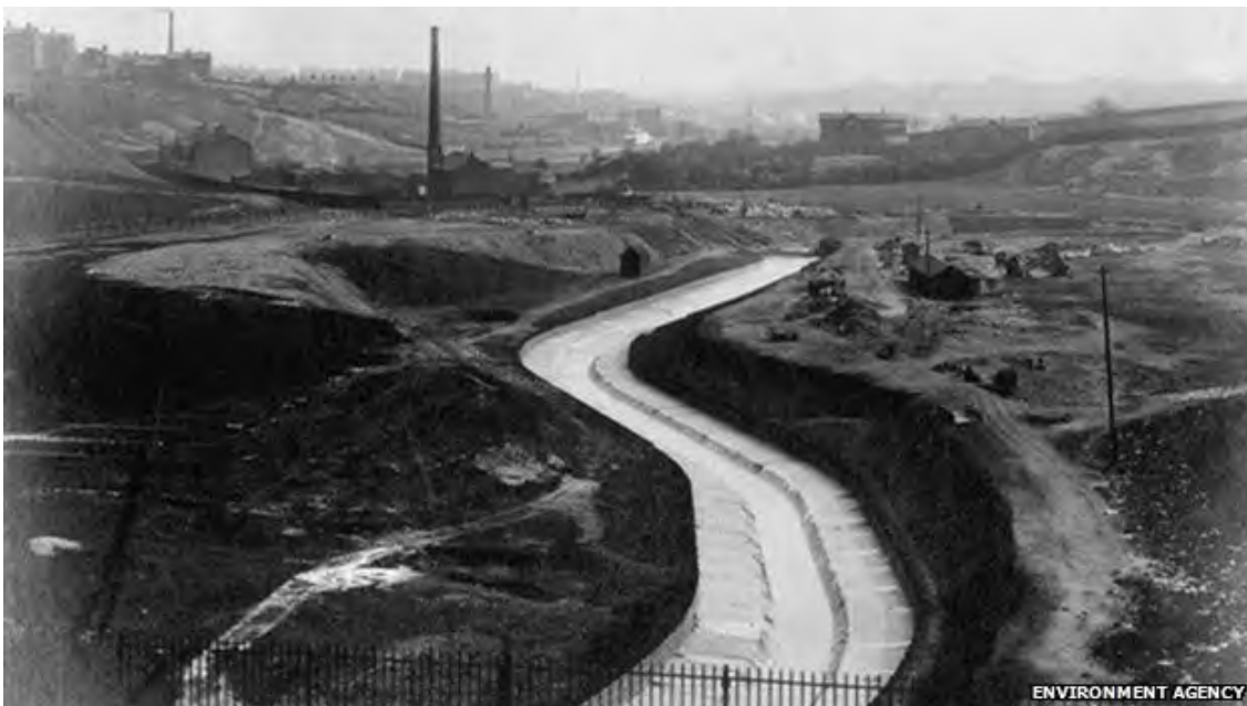
Figure 1—1 Historic brick channelled section of River Medlock upstream from Mayfield
