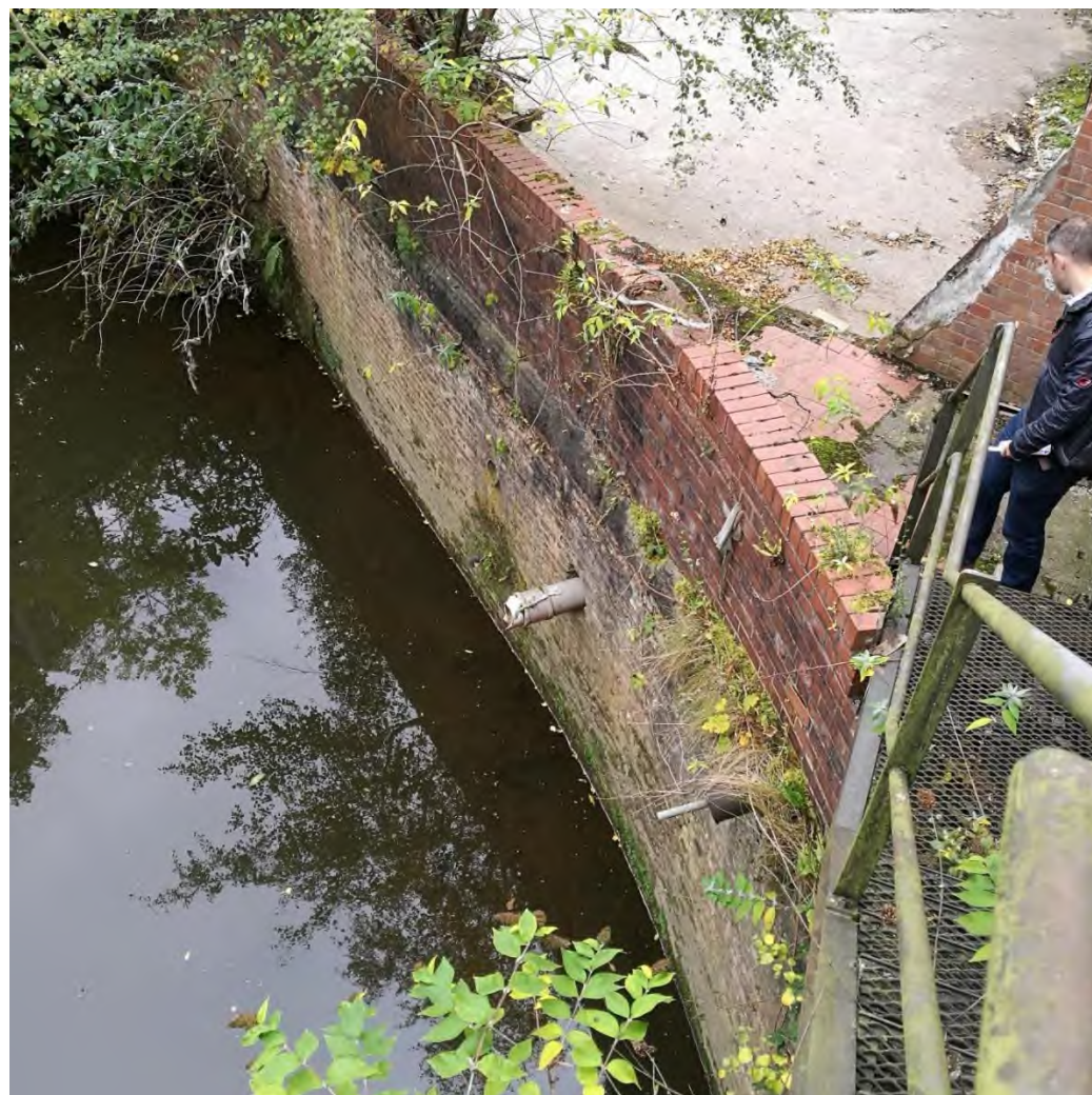
Figure 5-1 Existing Outfall Observed During Site Visit
