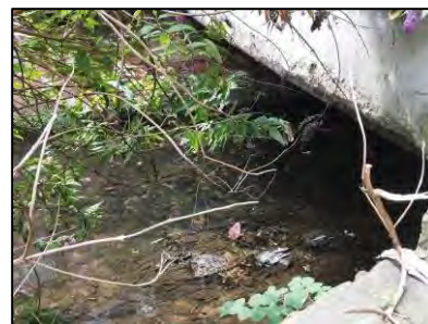
Entrance to culvert
