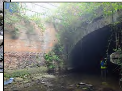
Upstream arched culvert
