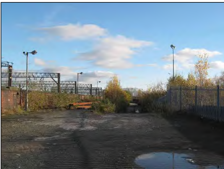
Plate 6 - Eastern section of the former railway station platform, looking east
