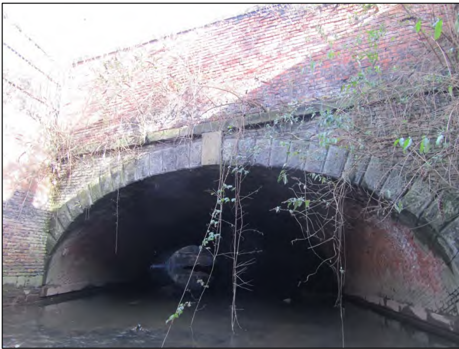
Plate 7 Culvert B26 looking upstream, showing on-site headwall. Brickwork largely intact with few crevices (February 2019)
