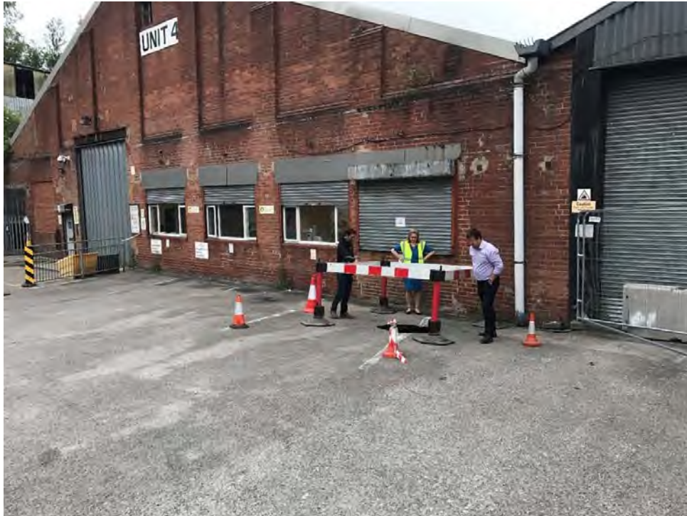
1. Location of void under car park
